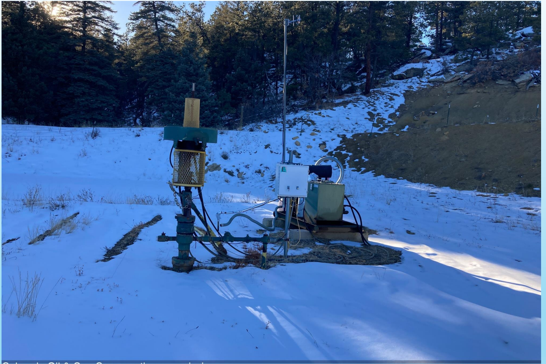
PHOTO 3: WELLHEAD AND EQUIPMENT
