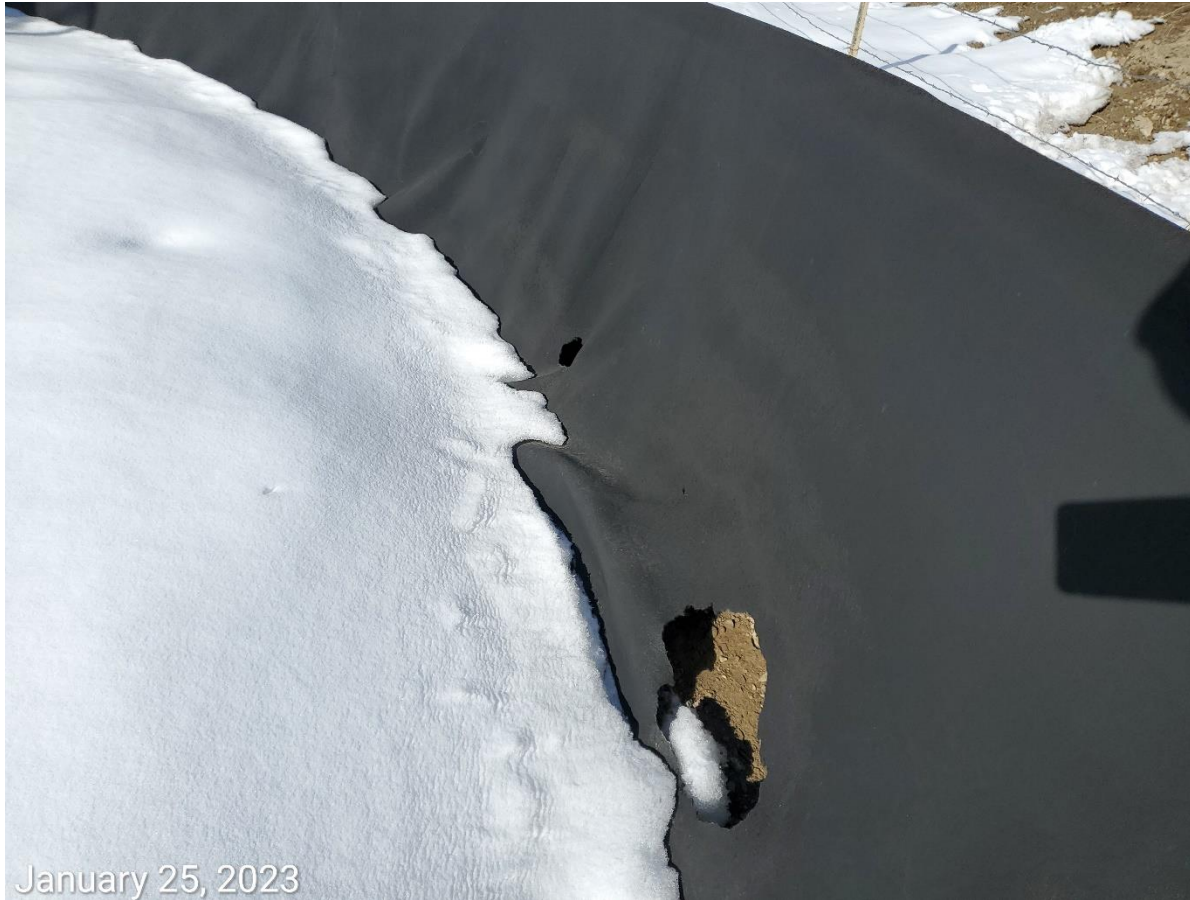
Photo 3: Photos 3-4 show holes observed within the secondary containment liner at the tank battery
