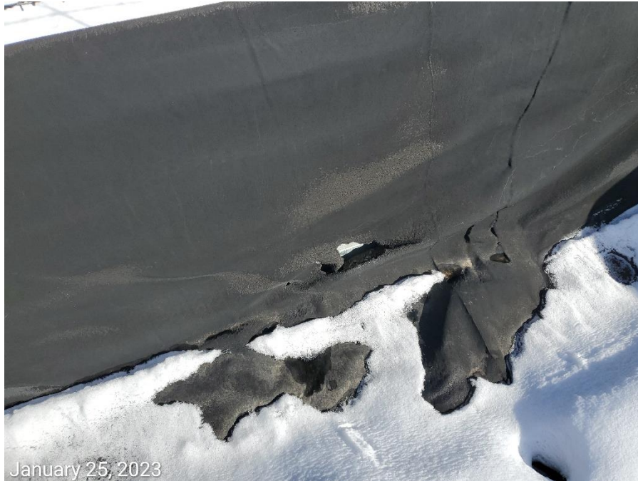
Photo 2: Photos 2-3 show holes observed within the secondary containment liner at the tank battery.
