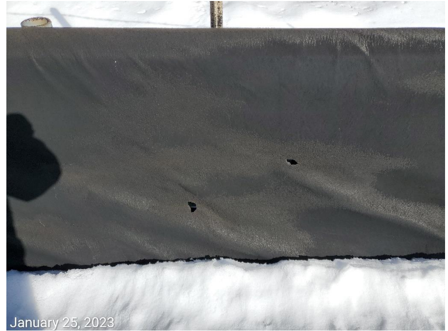
Photo 2: Photos 2-3 show holes observed within the secondary containment liner at the tank battery.
