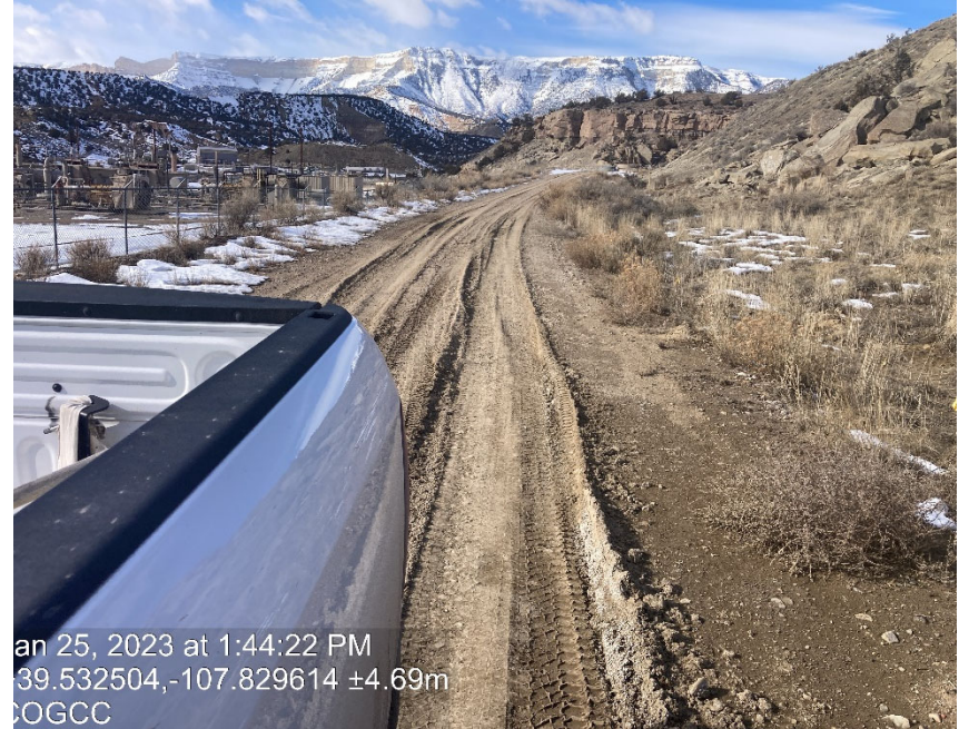
Access road lacks stabilization/compaction
