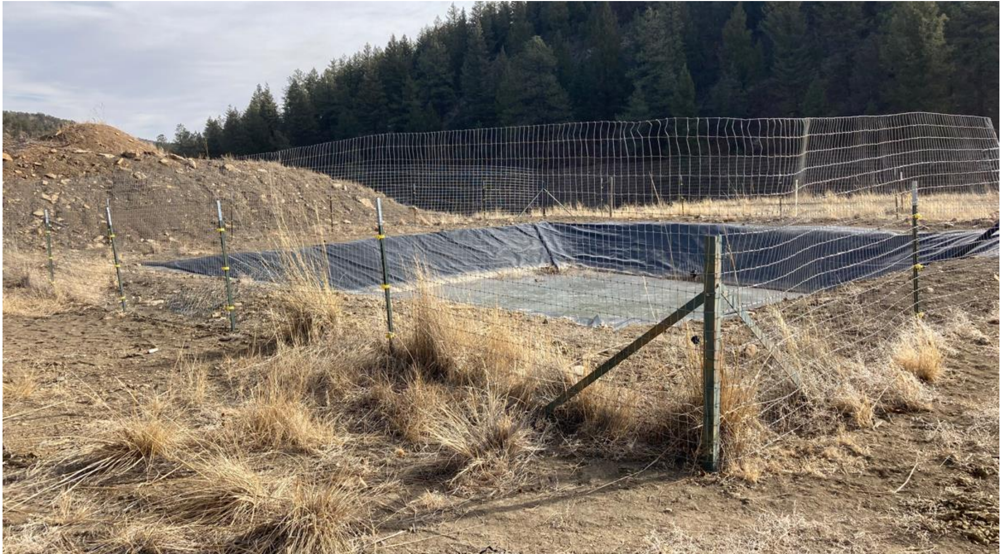
PHOTO 1: THE FENCING AROUND THE PIT HAS BEEN REPLACED TO COMPLY WITH 1002A RULES.
