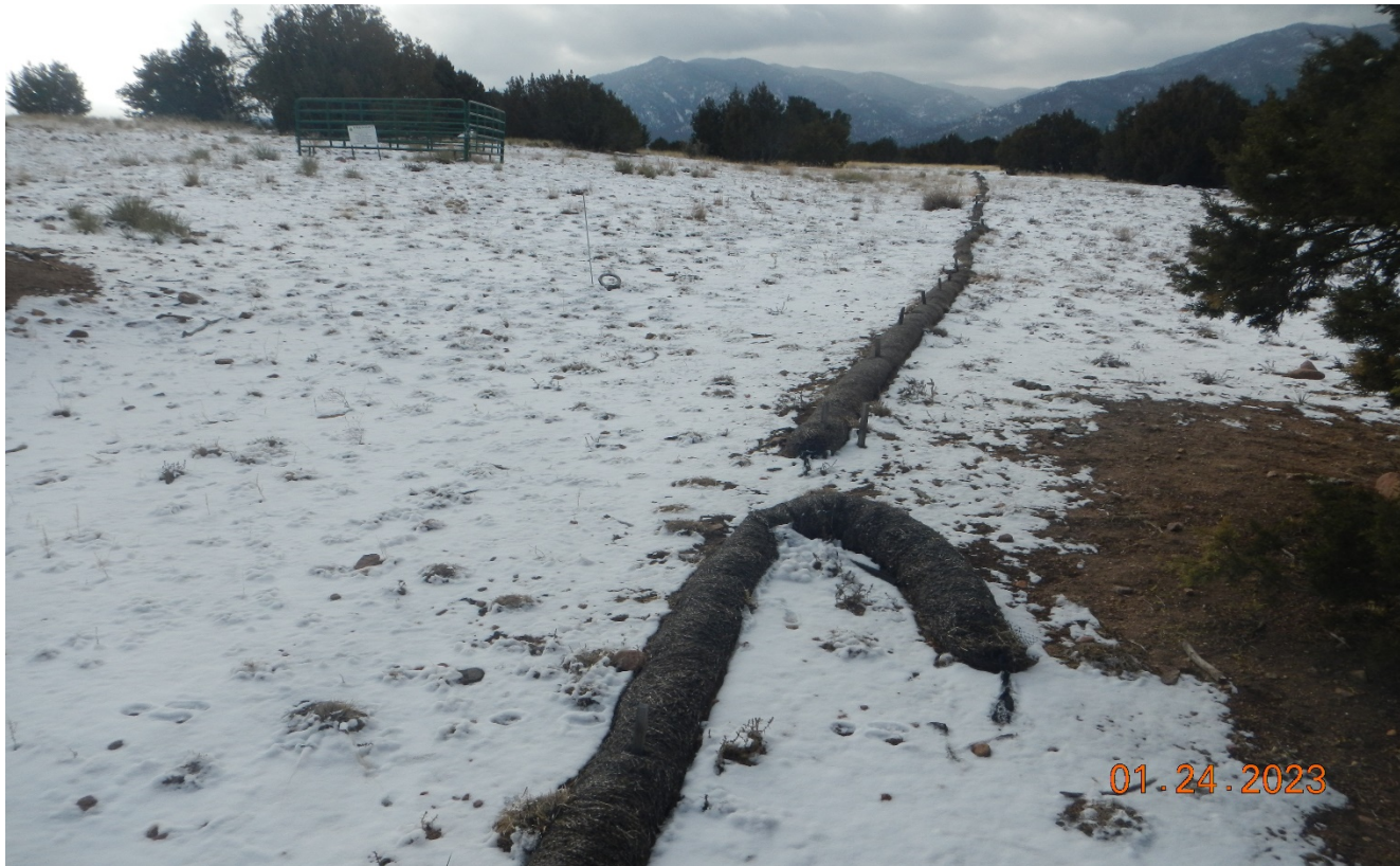
Photo 2. There are some degraded and displaced wattles that can be removed or replaced.
