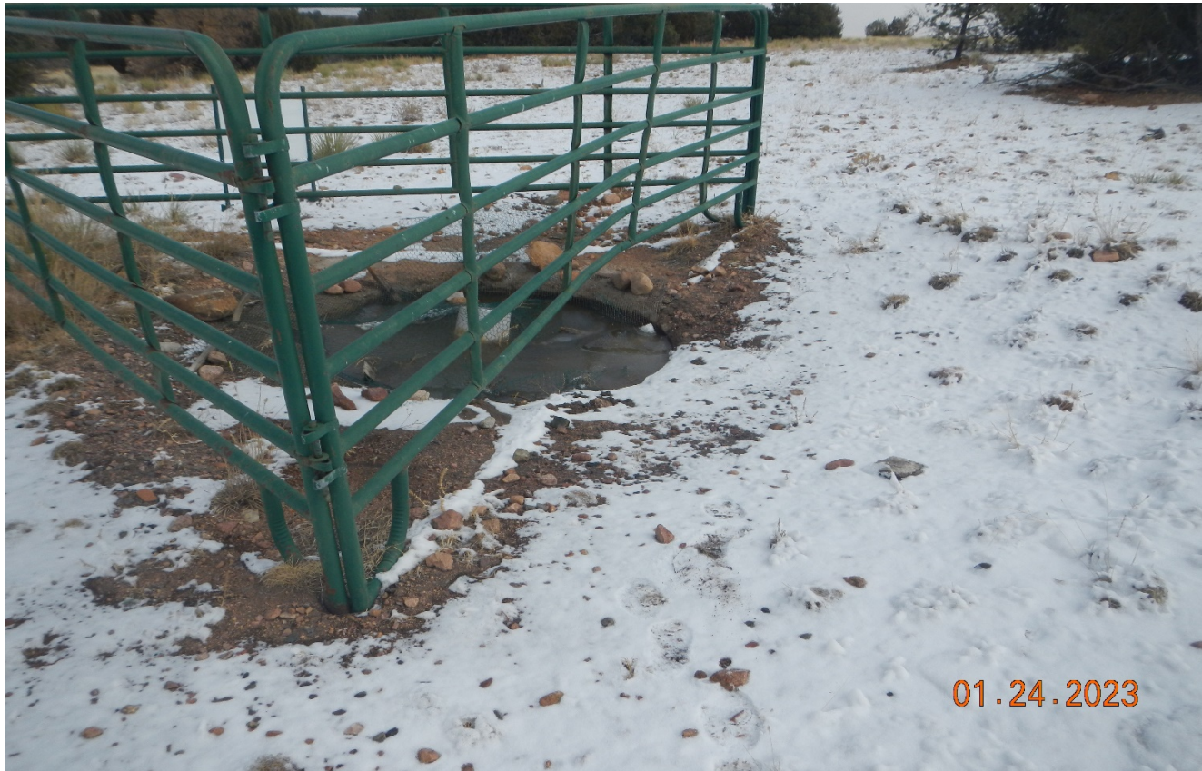
Photo 4. The panels have been moved and are not preventing access to the open cellar. The wire mesh over the cellar is also displaced.
