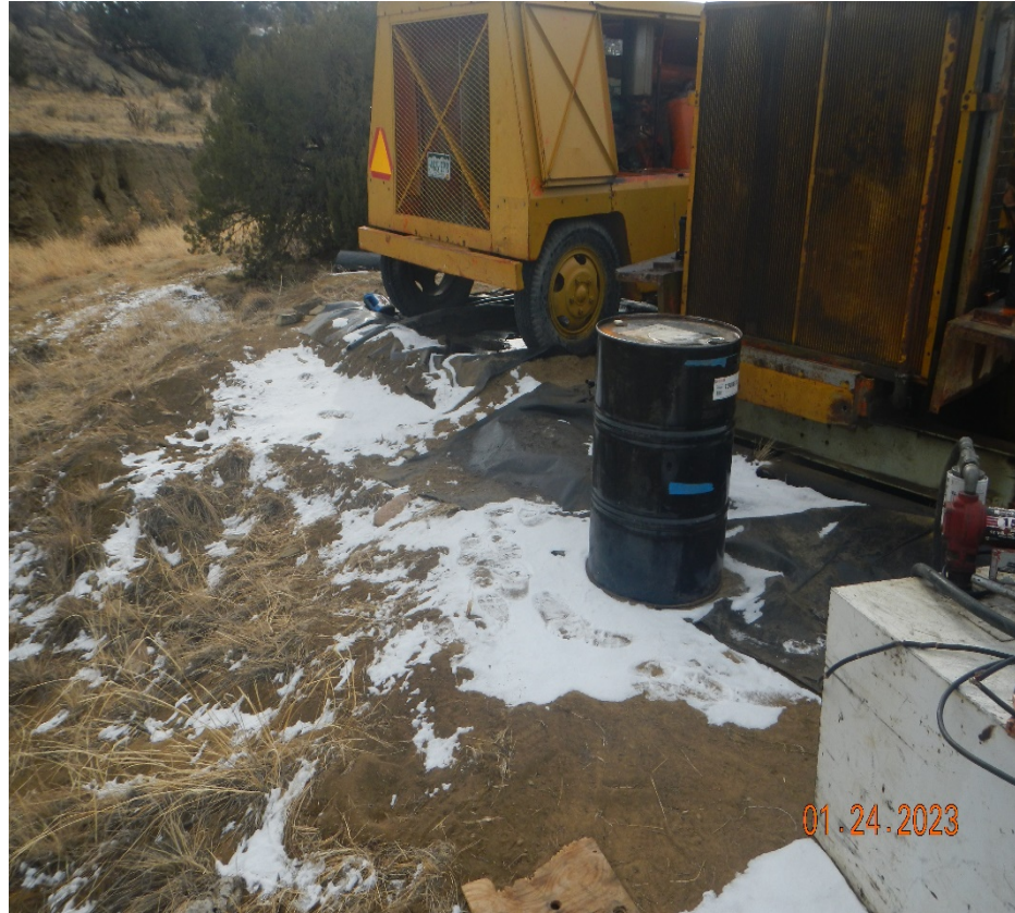
Photo 4. There is no down gradient perimeter controls toward the drainage in the left side of photo. This equipment is leaking fluids shown in the next two photos.
