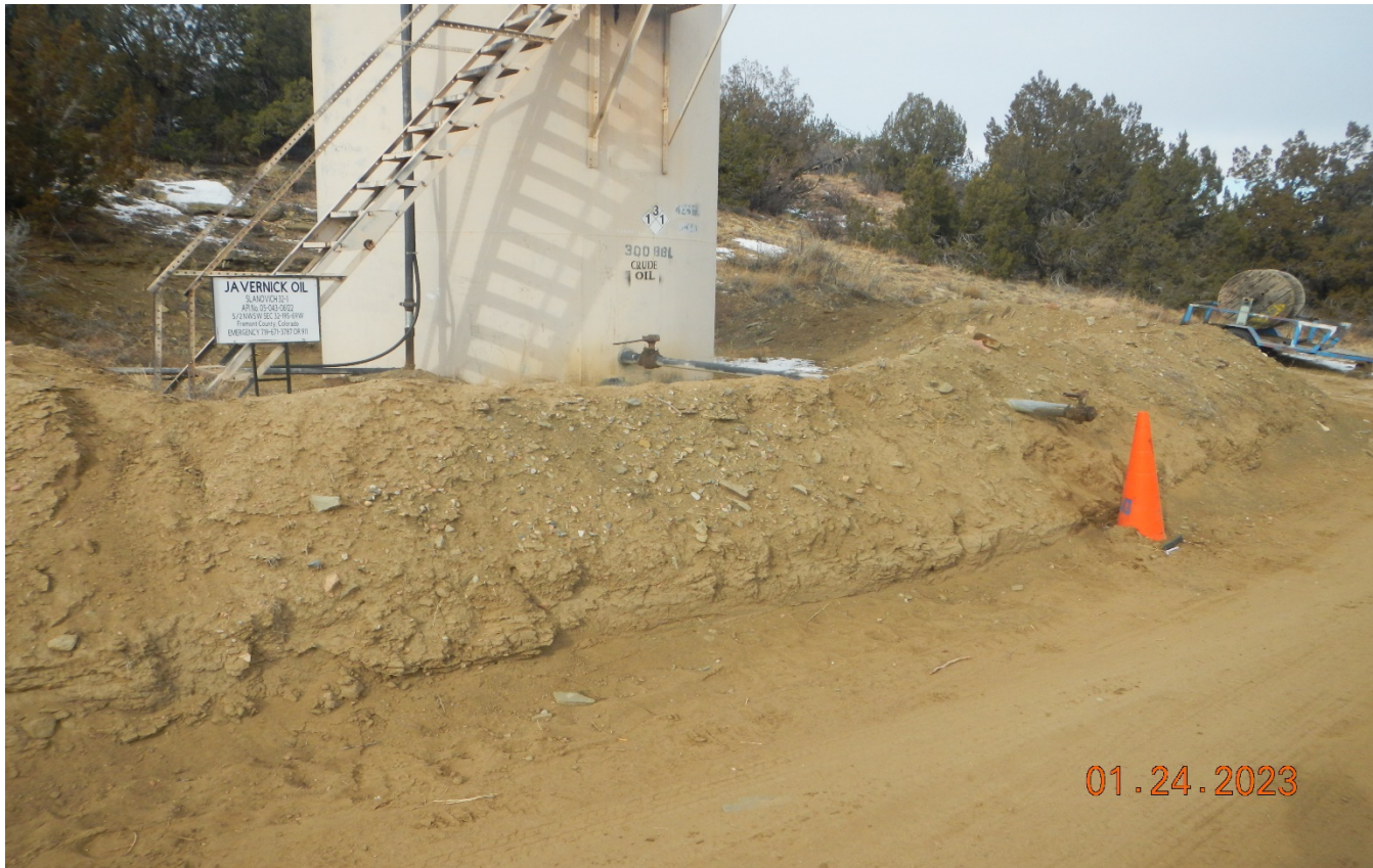
Photo 10. Facing toward the tank battery. There is still stained soils at the berm where the orange cone is located.
