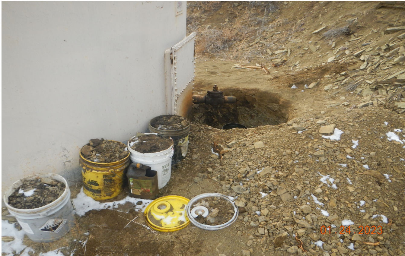
Photo 12. There are buckets of oily soils where it was excavated underneath the valve however the tank will likely need to be removed for further excavation.
