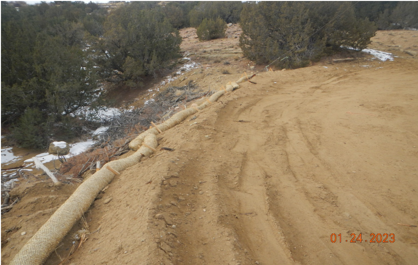
Photo 16. The wattle installed at the southern perimeter should have been position at the bottom of the slope to contain all loose soils that were pushed out and disturbed.
