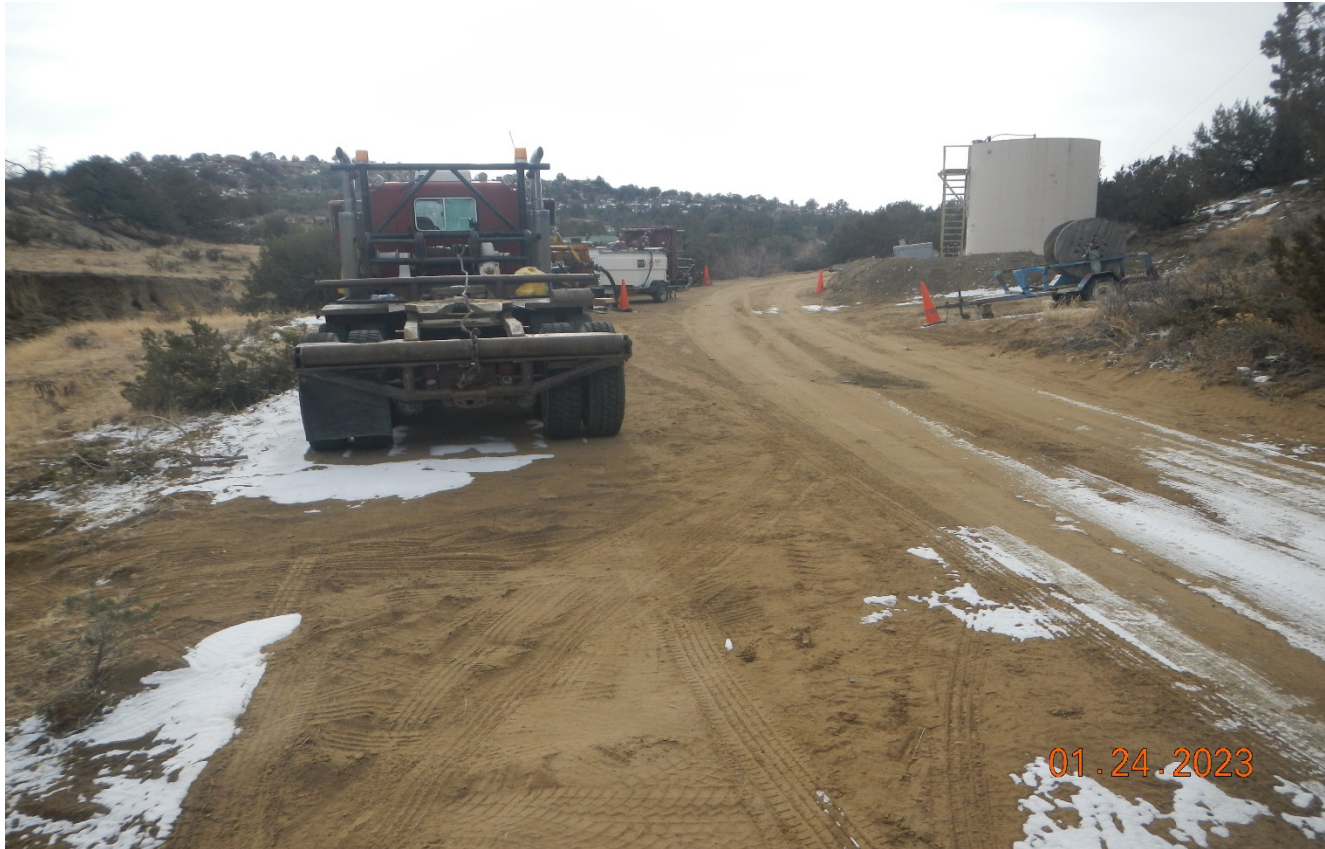
Photo 1. Facing southeast long the access road at the tank battery site. Soils were pushed out in this area toward the drainage and no BMP's along down gradient perimeter. Drilling equipment is being stored in this area.
