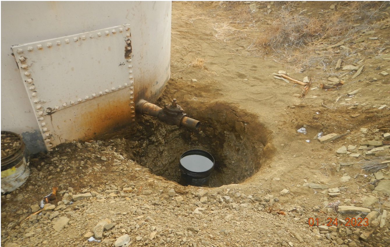
Photo 11. There is a dripping leak at the backside valve and the 5 gallon bucket is filled with oil. There is oil stained soils underneath the tank. Tank may need to be removed to cleanout the contaminated soils. This needs to be cleaned up immediately.
