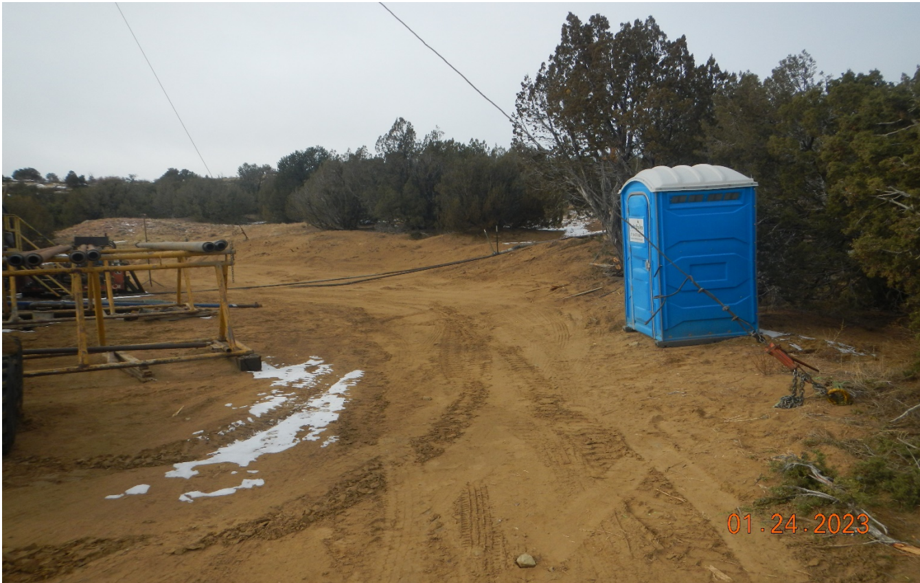
Photo 21. Facing southwest at the location. The portable outhouse was not staked down and could fall over. There are no run-on stormwater controls along the west side of the location.
