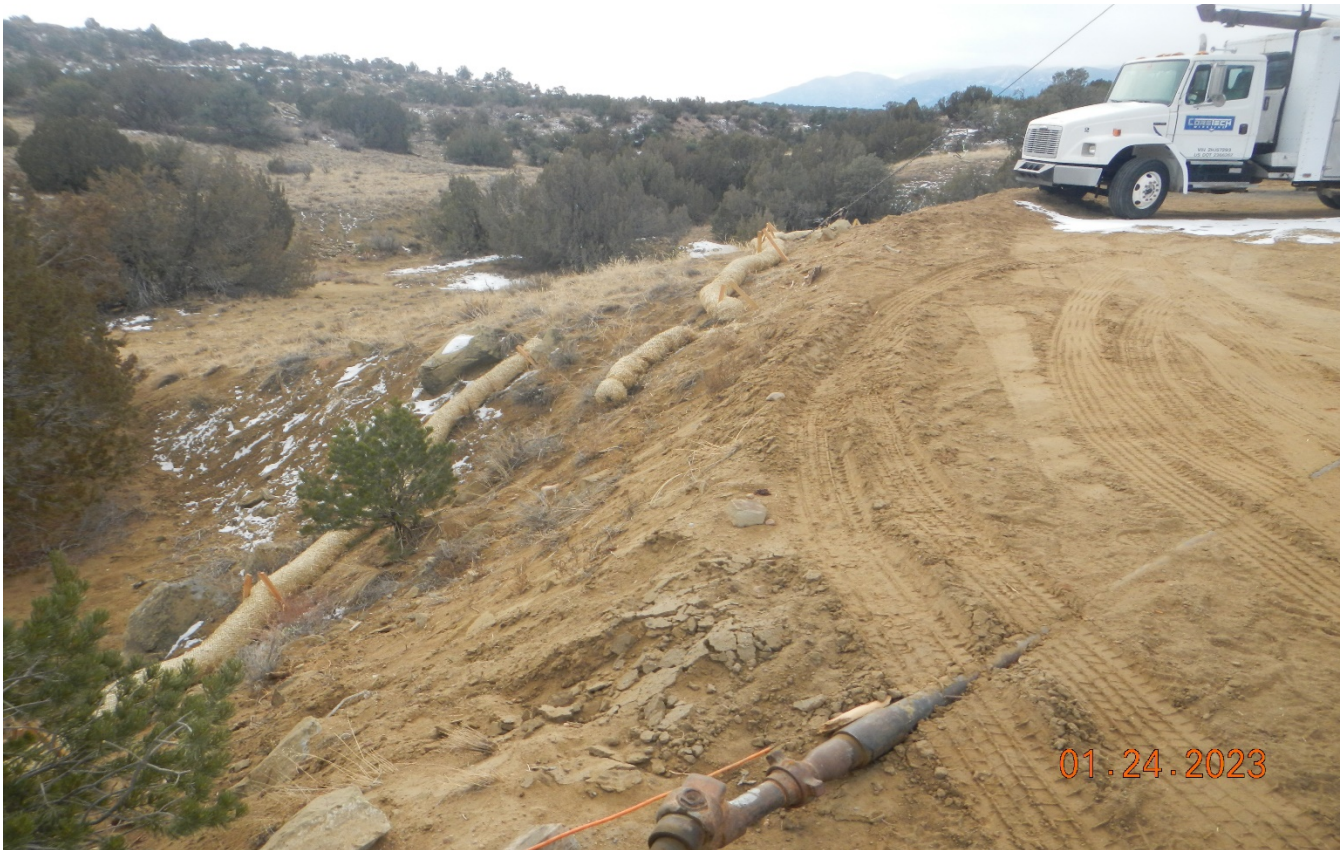
Photo 14. Facing southeast along the fill slope of the pad. There are wattles installed however they are not properly installed per good engineering practice. Wattles are not properly positioned, trenched, or staked down.
