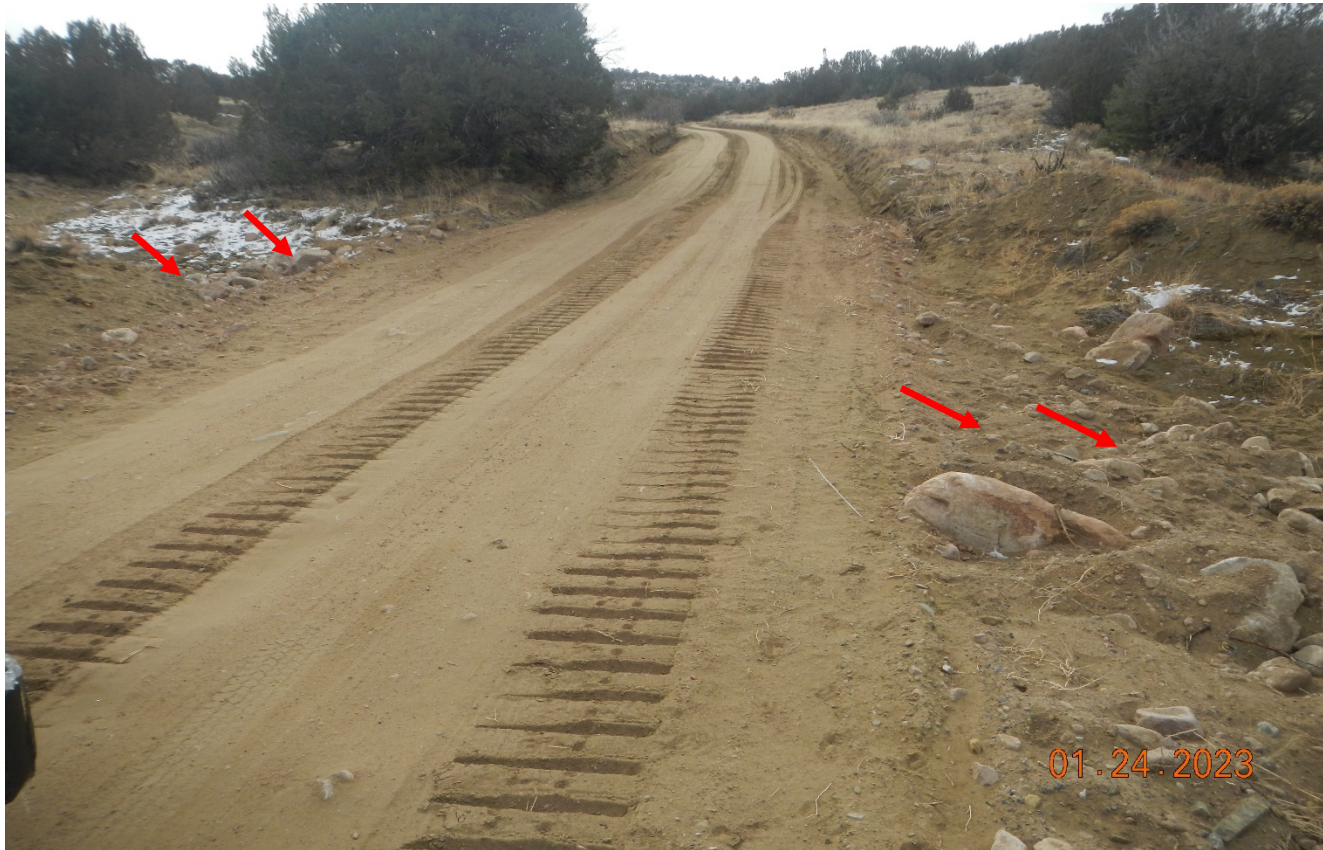
Photo 1. Facing southeast long the access road. This drainage crossing must have BMP's installed to accommodate seasonal storm event to prevent material from washing out. BMP may include culvert, rip/rap, ect. Previous corrective action not completed. Red line shows direction of drainage flow.
