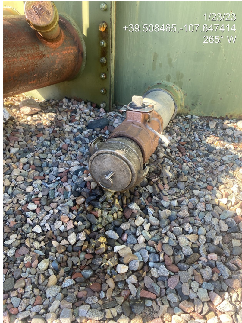
Photo 3. Photo shows staining beneath a produced water/condensate tank drain line.
