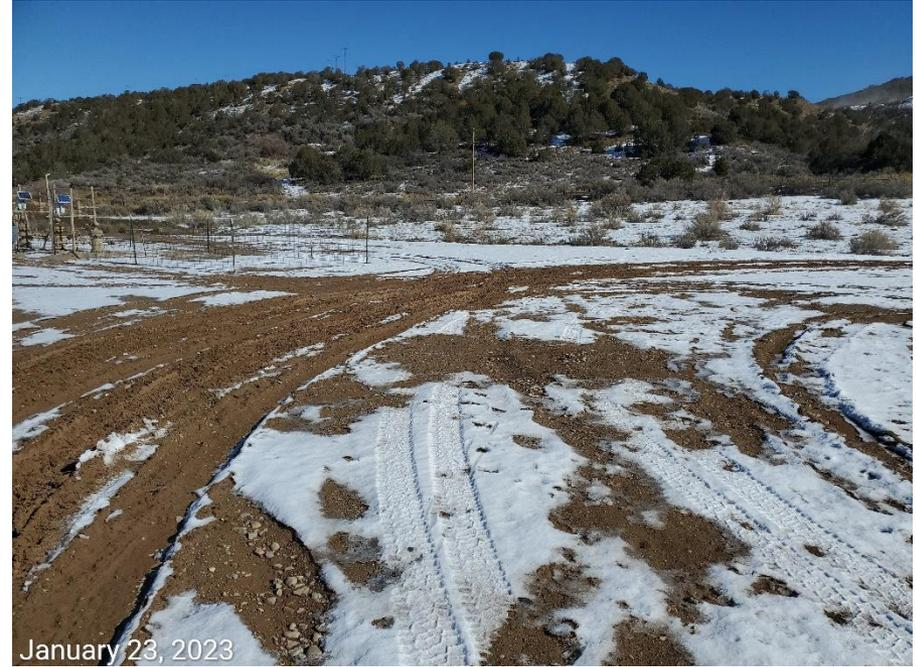
**Photo 1:** Photos taken from the west end of the Location, facing north. Photos 1-4 provide an overview of the Location from north, northeast, southeast to south. Photos 1-3 also show that BMPs to stabilize the Location, and to minimize degradation, tracking and sediment transport from the working pad areas are missing or insufficient.
