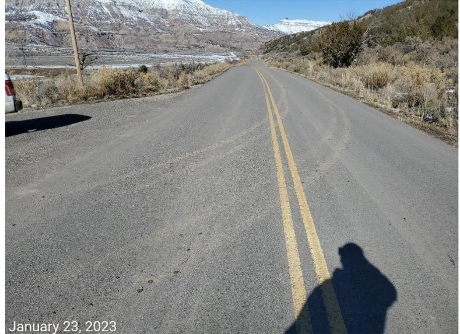
**Photo 4:** Photos taken from the access road entrance point from Stone Quarry Road. Photo shows sediment transport via vehicle tracking from the Location onto the county road.
