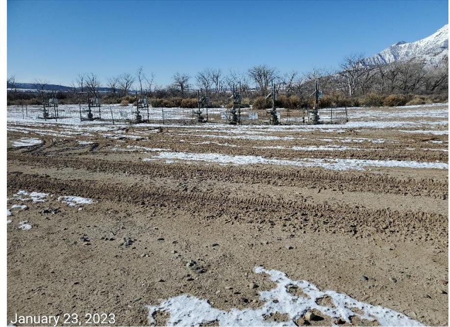
**Photo 1:** Photos taken from the east end of the Location, facing south. Photos 1-2 provide an overview of the Location from south, southwest, northwest to north. Photos 1-3 also show that BMPs to stabilize the Location, and to minimize degradation, tracking and sediment transport from the working pad areas are missing or insufficient.
