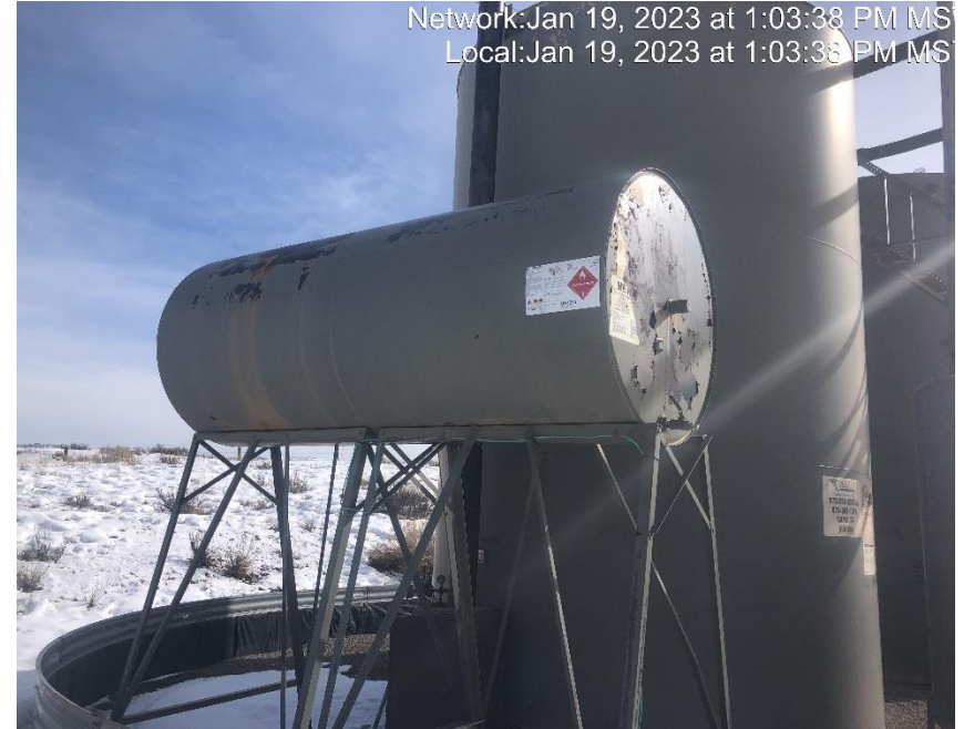
Photo #8821 Methanol tank missing required information.
