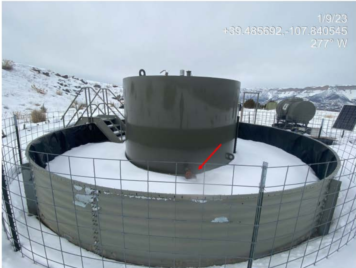
Photo 2. Photo shows a bull plug is not installed on the tank drain .
