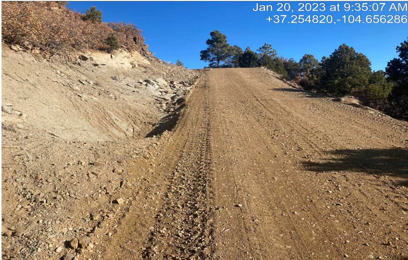
Photo 2. Facing northeast along the main access road past the compressor. The roadside was repaired and BMP maintenance was performed.
