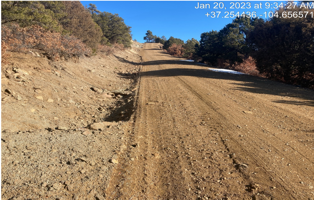
Photo 1. Facing northeast along the main access road past the compressor. The roadside was repaired and BMP maintenance was performed. Additional road base was applied to the road.
