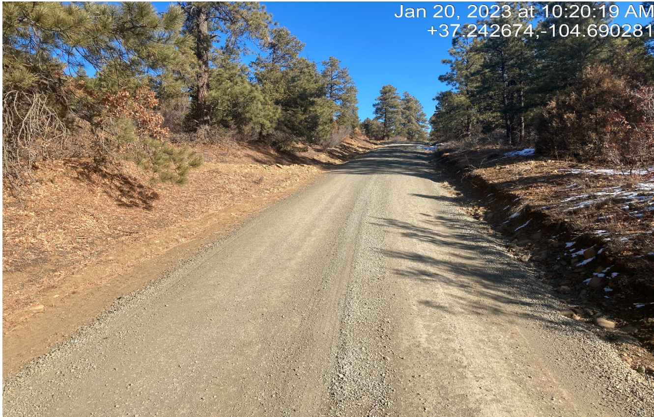
Photo 3. Facing northeast along the main access road. BMP's appear to be maintained along the road and additional road base was applied to this steep area for stabilization.
