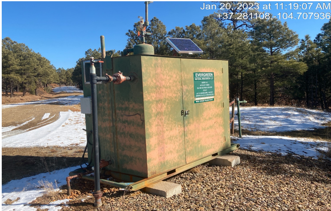
Photo 2. Well sign is posted on back side of meter shed and should be relocated to a more conspicuous place.
