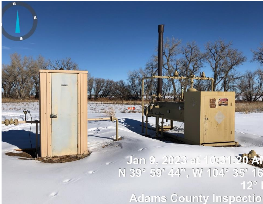
Photo#3 Gas Meter/Separator
