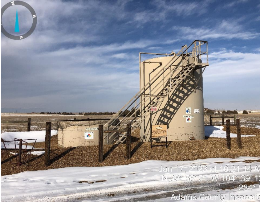
Photo# 1 Crude & P/W tanks.
