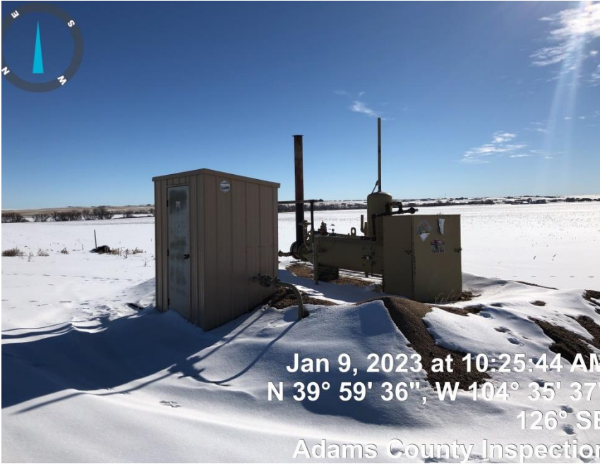
Photo#2 Gas Meter/Separator
