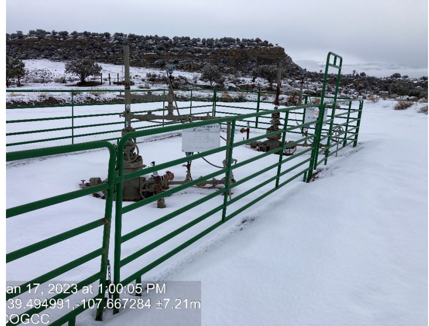
Signage is faded and illegible
