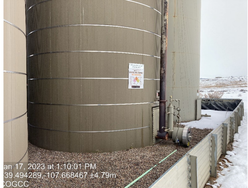
Tank label illegible quantity
