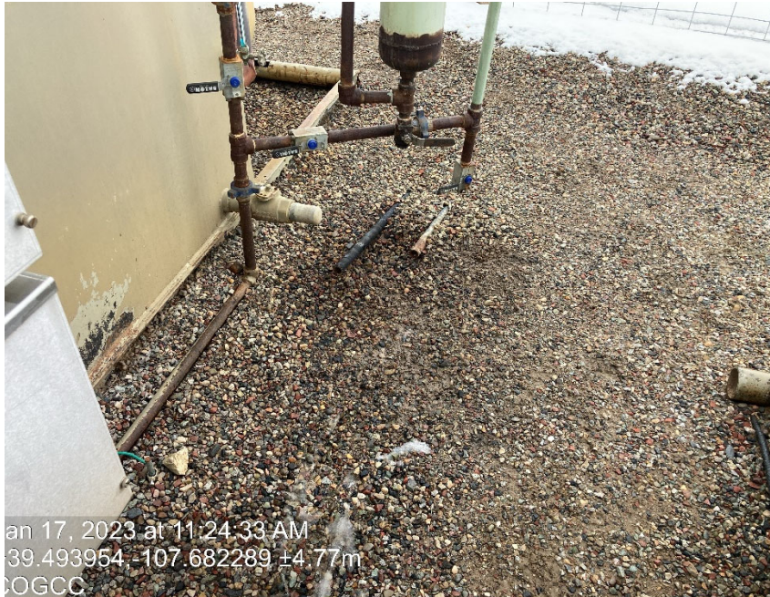
Staining under knock out pot
