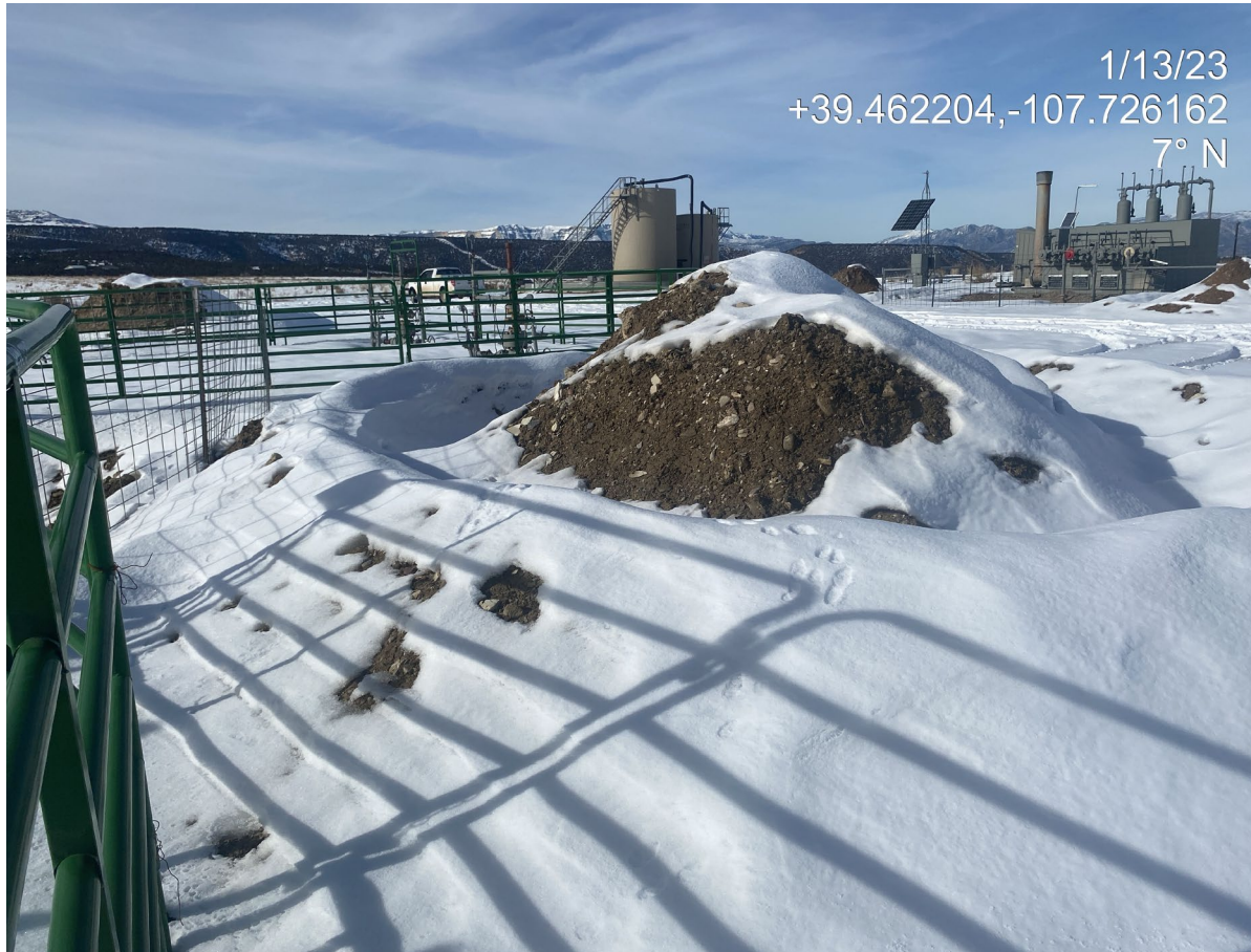
Photo 2. Photo shows stockpiled soil associated with plugged and abandoned well API #045-09126. Perimeter control berm does not appear properly compacted. Soils are loose, and susceptible to wind and water erosion and may act as a sediment source.
