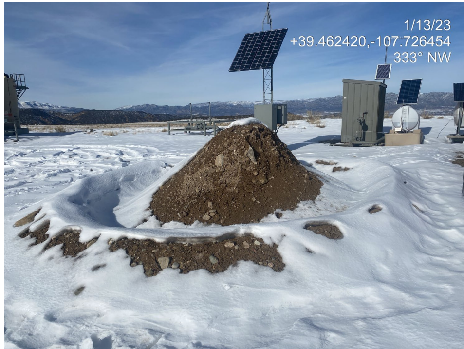
Photo 4. Photos show stockpiled soil associated with plugged and abandoned well API #045-09128 (left) and the associated separator and flowline (right) excavations. Perimeter control berm does not appear properly compacted. Soils are loose, and susceptible to wind and water erosion and may act as a sediment source.
