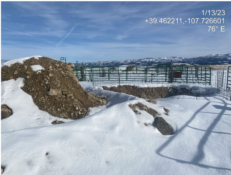
Photo 4. Photos show stockpiled soil associated with plugged and abandoned well API #045-09128 (left) and the associated separator and flowline (right) excavations. Perimeter control berm does not appear properly compacted. Soils are loose, and susceptible to wind and water erosion and may act as a sediment source.
