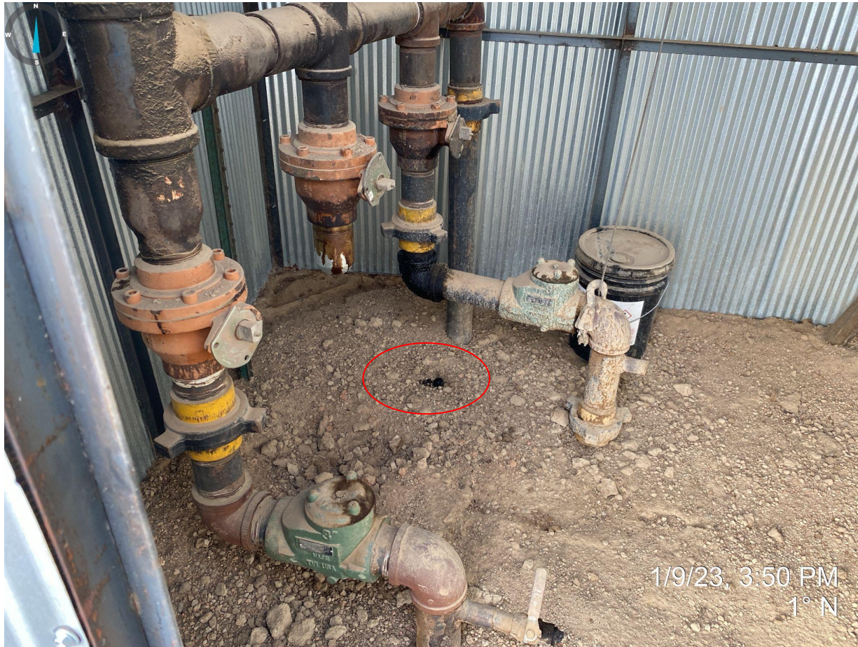
Photo 7. Facing north from inside of shed, north of skim pit. Photo illustrates oil stained soils coming from a leaky fitting.
