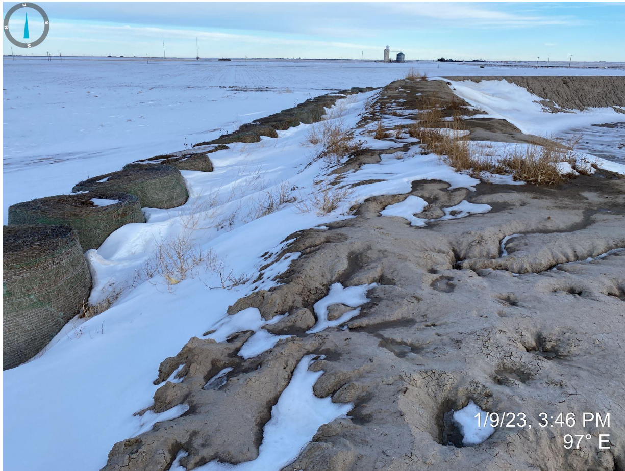
Photo 11. Facing east from the northeastern corner of pit. Photo illustrates undesirable weedy vegetation (e.g. russian thistle and kochia); this is now considered debris and needs to be removed.
