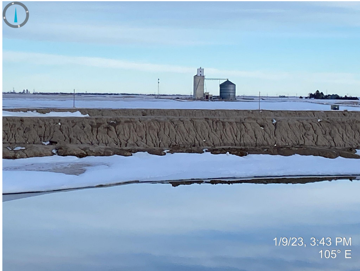
Photo 8. Facing east from skim pit. Photo illustrates rill erosion occurring on the interior pit wall; these walls are not stabilized as the material is unconsolidated.
