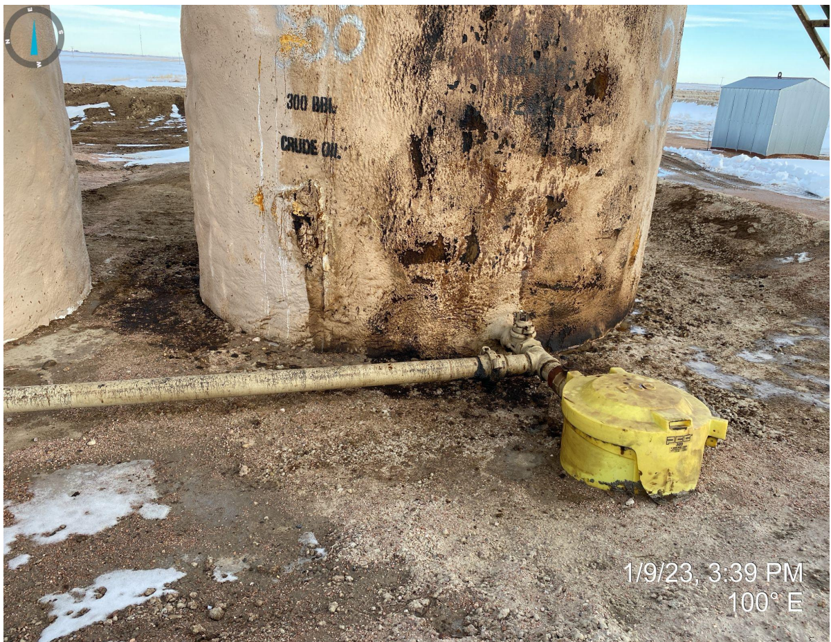
Photos 3 & 4. Facing east at tank battery. Photos illustrates crude oil spill appearing to come from the top of the tank near the thief hatch. Also pictured, oil stained soil around the bottom of the tank.
