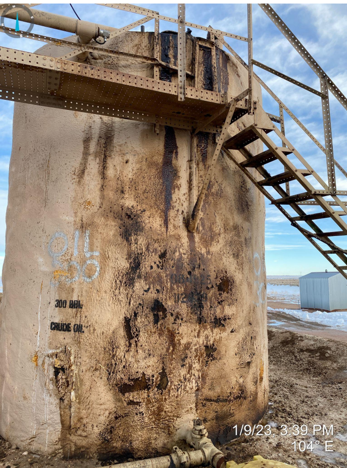
Photos 3 & 4. Facing east at tank battery. Photos illustrates crude oil spill appearing to come from the top of the tank near the thief hatch. Also pictured, oil stained soil around the bottom of the tank.
