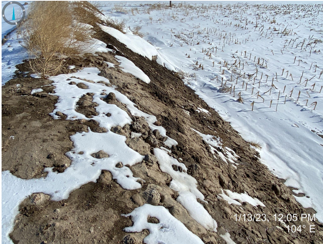
Photo 7. Facing east from southern pit wall. Photo illustrates the pit wall is unstabilized with evidence of rill erosion and unconsolidated material. These walls need to be repaired/stabilized to prevent further erosion from migrating off location.
