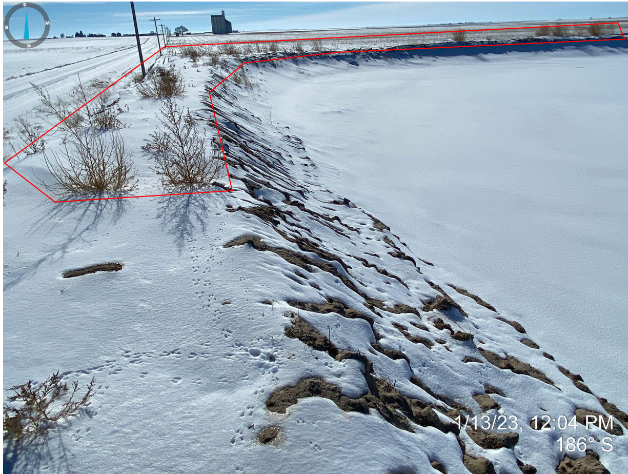
Photo 5. Facing south from the eastern pit wall. Photo illustrates rill erosion and unconsolidated material comprising the interior walls; e.g. not stabilized. Also pictured, undesirable weedy vegetation (e.g. kochia and russian thistle) that is considered debris and needs to be removed and managed for in the future.
