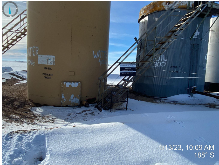
Photos 1 & 2. Facing south and southeast at tank battery. NFPA placards are missing and or not legible.
