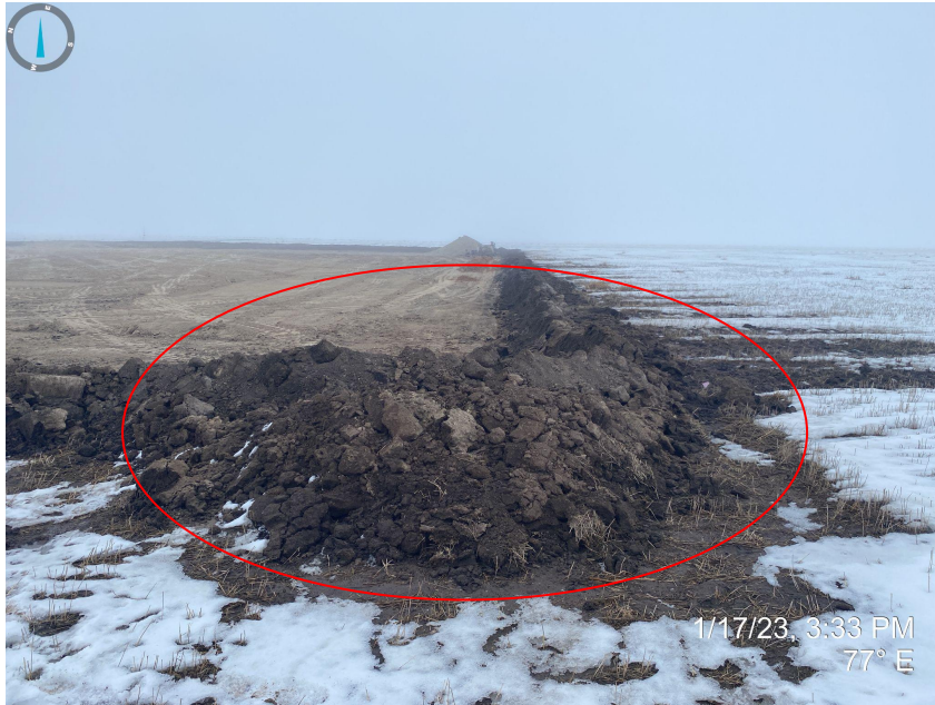
Photos 9 & 10. Facing east (photo 9) and north (photo 10) from the southwestern portion of the location. Photo illustrates that portions of the perimeter berm/BMP are comprised of unconsolidated material and not properly stabilized.
