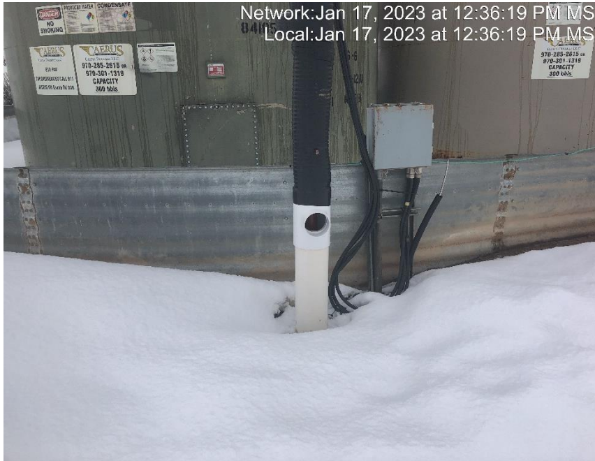
Photo #8802 Flowline heating insulation open ended.
