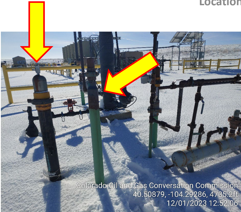
Photo 13 – Unmarked Riser
