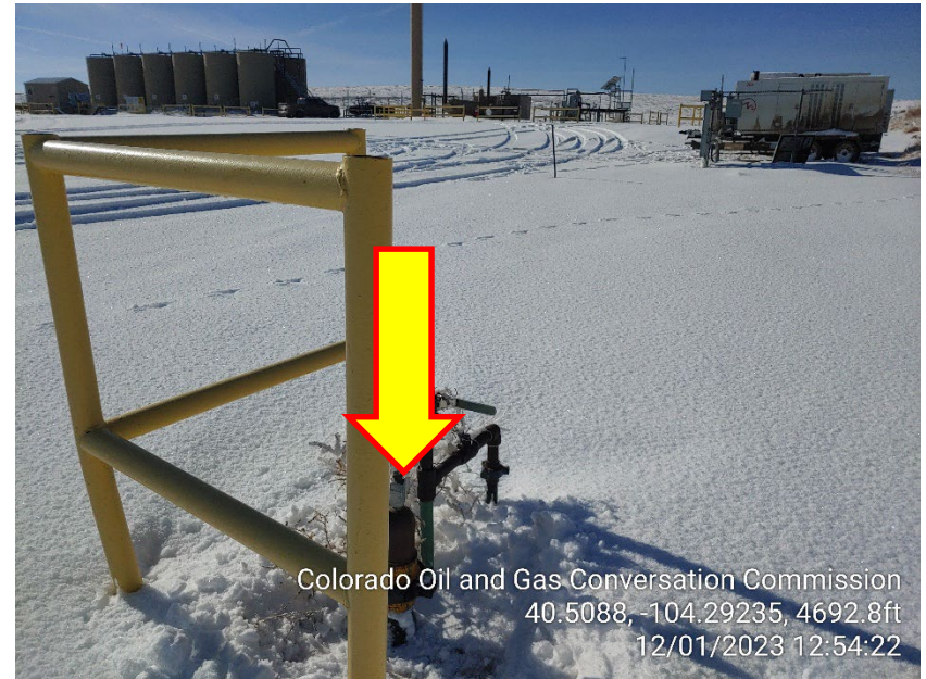
Photo 12 – Unmarked Riser
