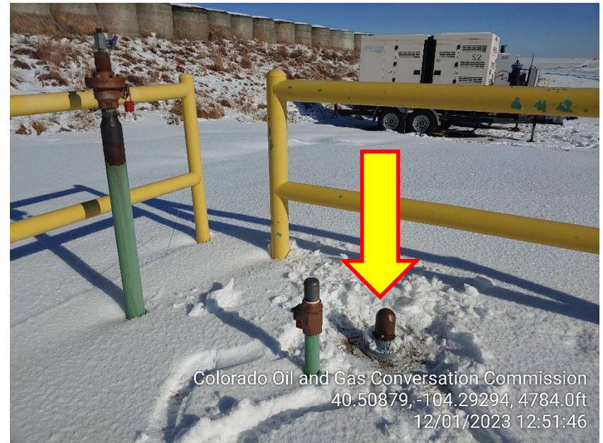
Photo 10 – Unmarked Riser
