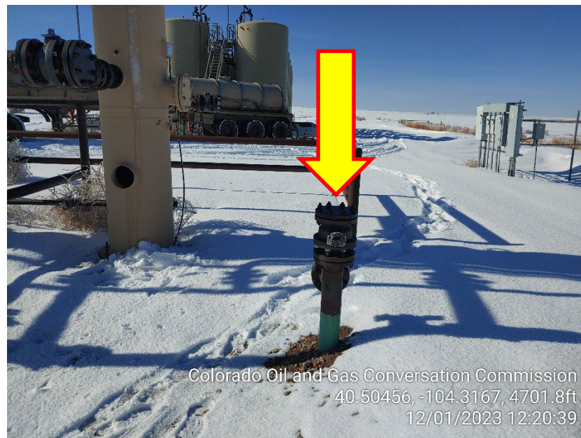
Photo 8 – Unmarked Riser
