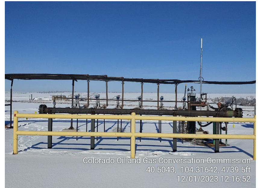
Photo 4 – Gas Lift Injection Meters
