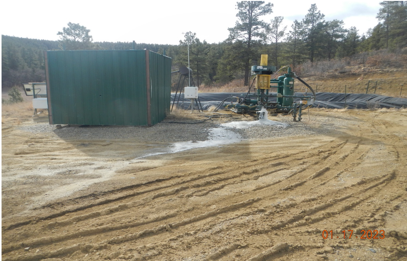
Photo 2. There is a dripping leak at the wellhead that needs to be repaired.
