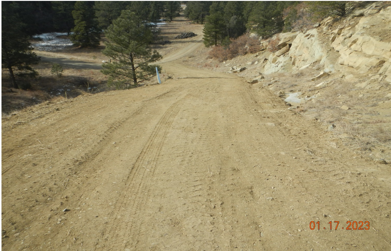
Photo 2. Facing back down the steep portion of the road. BMP's need to be installed to prevent erosion which may include road base, water bars, check dams ect.
