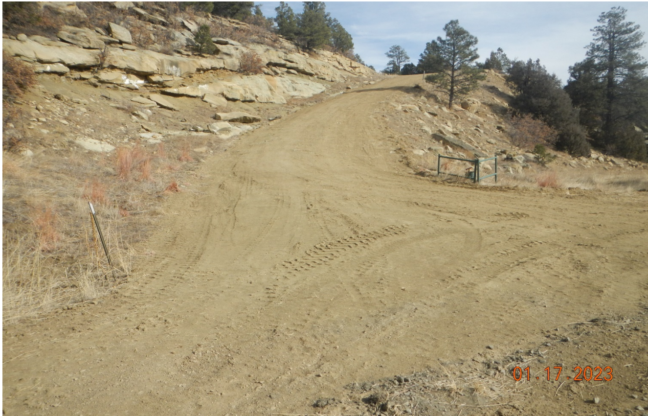
Photo 1. Facing at the beginning of the access road. The road was regraded however there was no BMP's installed to prevent erosion from reoccurring. Grading has caused disturabce which needs to be stabilized.
