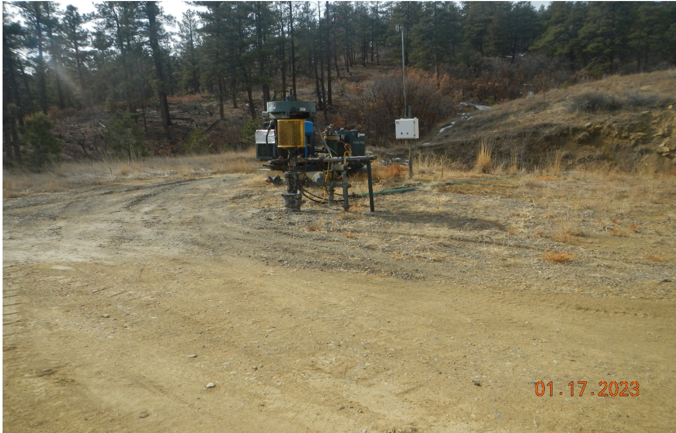
Photo 2. Leak at wellhead was repaired.
