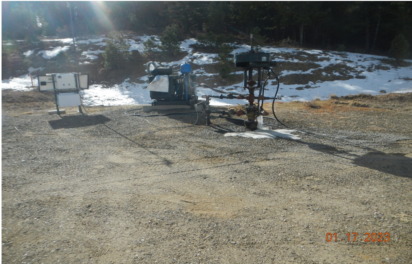
Photo 3. There is a dripping leak at the wellhead that needs to be repaired.
