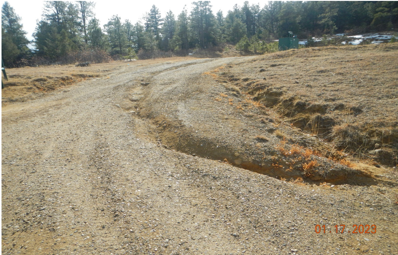
Photo 1. There is erosion along the access road near the location which needs to be repaired.
