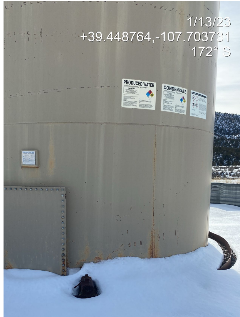
Photo 2. Photo shows a bull plug is not installed on the tank drain line.
