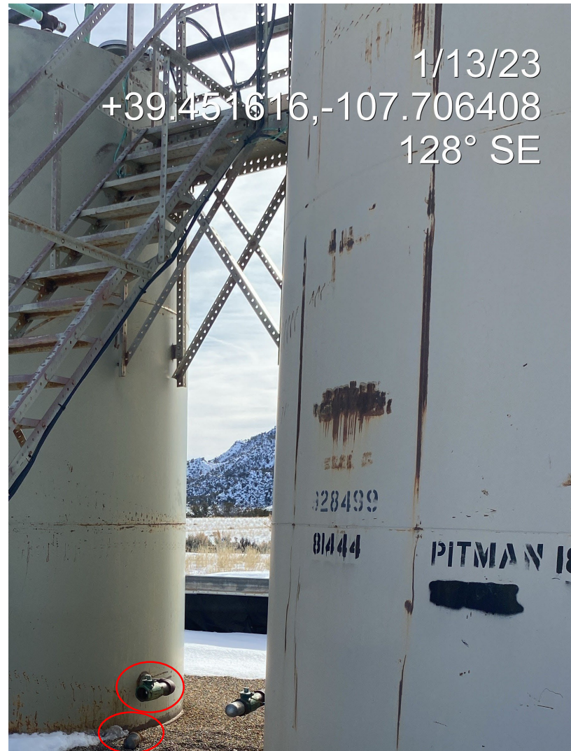
Photo 2. Photo shows a bull plug not installed on a tank drain line.
