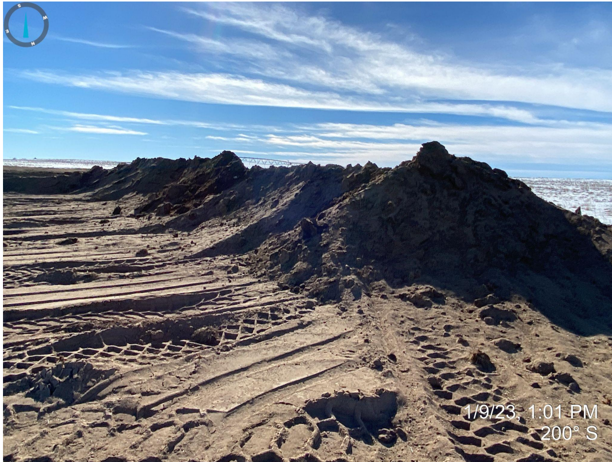
Photo 3. Facing south near one of the topsoil stockpiles on the west end of the location. Photo illustrates this stockpile has not been stabilized with no evidence of temporary equipment tracking and unconsolidated material present. Tires tracks are from a loader grabbing soil from the stockpile and is not considered a temporary BMP.
