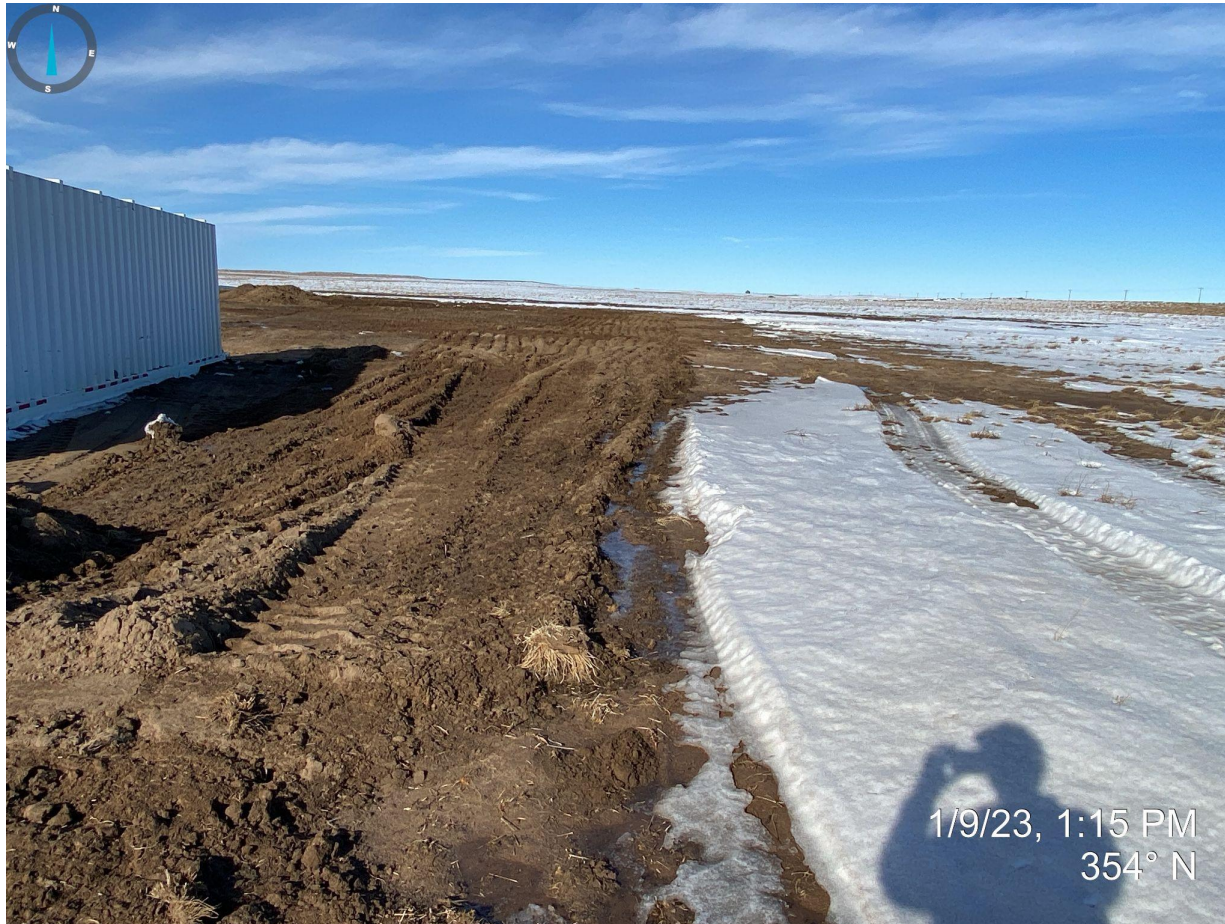
Photo 8. Facing north from the southeast corner of the location. Photo illustrates no stormwater controls/BMPs are installed to prevent sediment laden stormwater from exiting off location. This is the downslope/gradient side of the location. Stormwater controls should be implemented and installed until final reclamation has been achieved.
