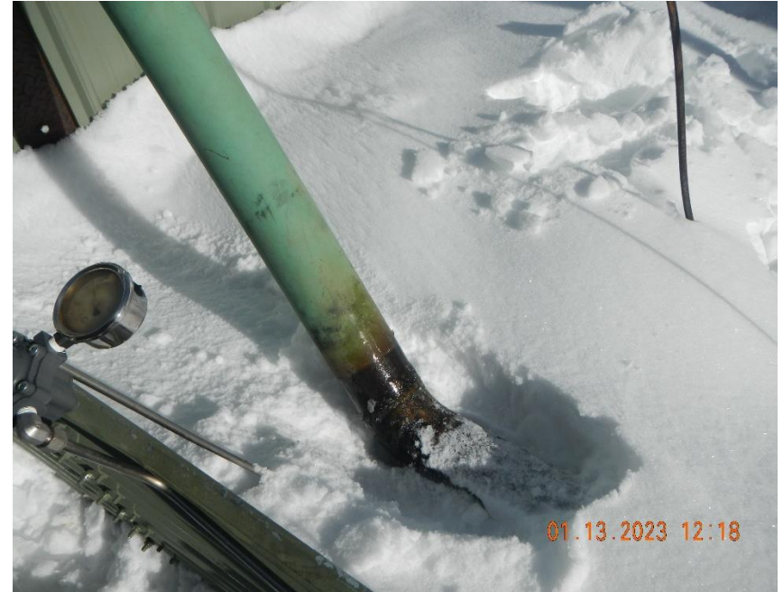
Replaced section of suction line.
