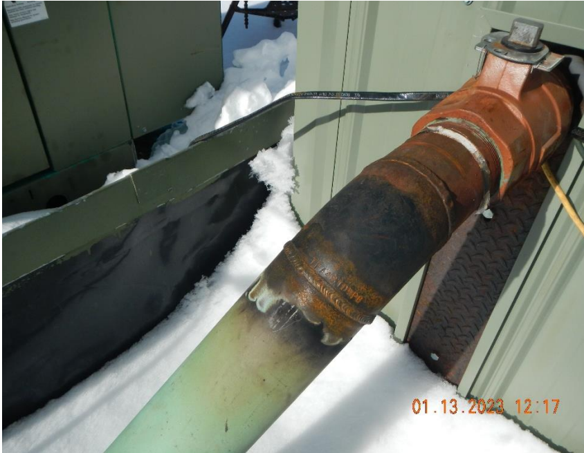
Replaced section of suction line.
