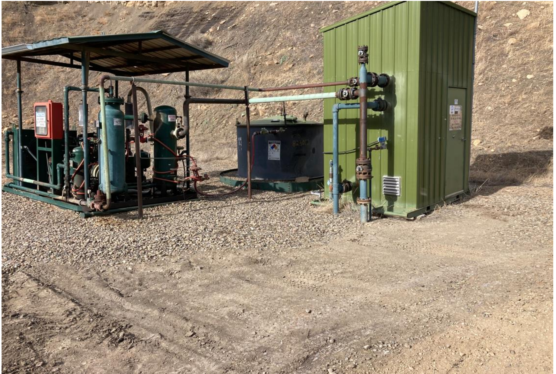
PHOTO 3: THE LEAK AT THE METER SHED HAS BEEN REPAIRED, IMPACTED SOIL HAS BEEN REMOVED AND PROPERLY DISPOSED. ALL VALVES, PIPES AND FITTINGS ARE SECURLY FASTENED AND THE SELF INSPECTION PROCESS HAS BEEN REVIEWED.
