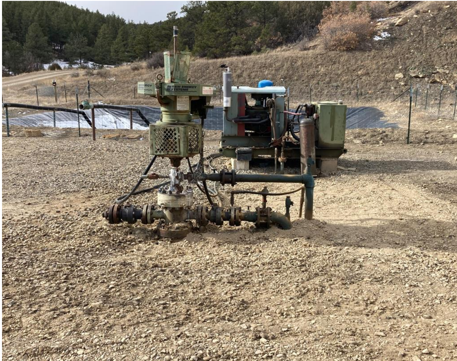
PHOTO 2: THE IMPACTED SOIL AT THE WELL HEAD HAS BEEN REMOVED AND PROPERLY DISPOSED IN ACCORDANCE WITH THE OGRIS OPERATING WASTE MANAGEMENT PLAN. MAINTENANCE HAS BEEN PERFORMED AND THE SELF INSPECTION PROCESS HAS BEEN REVIEWED.
