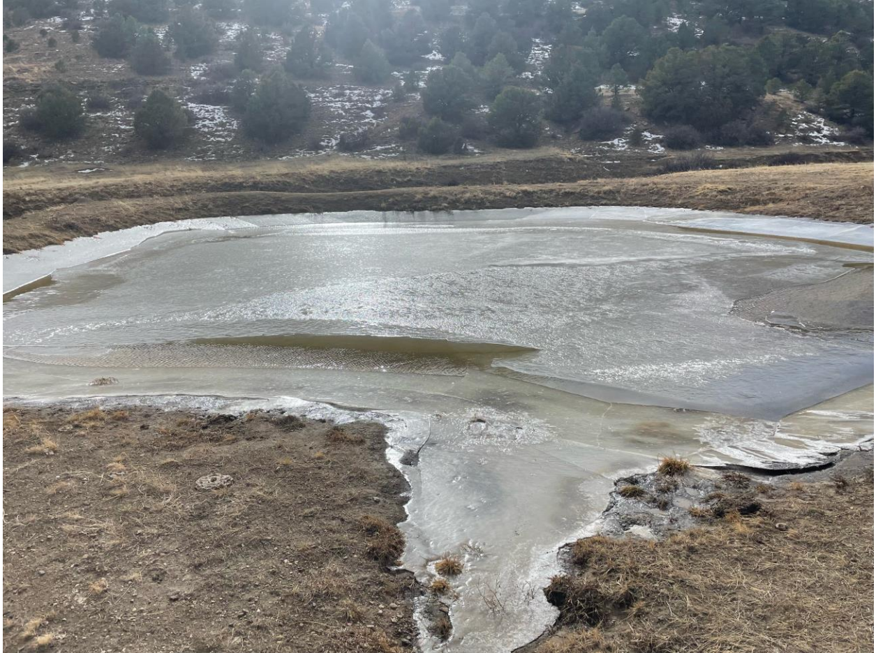
Lowered fluid level so two feet of freeboard exist per Rule 909.c.
