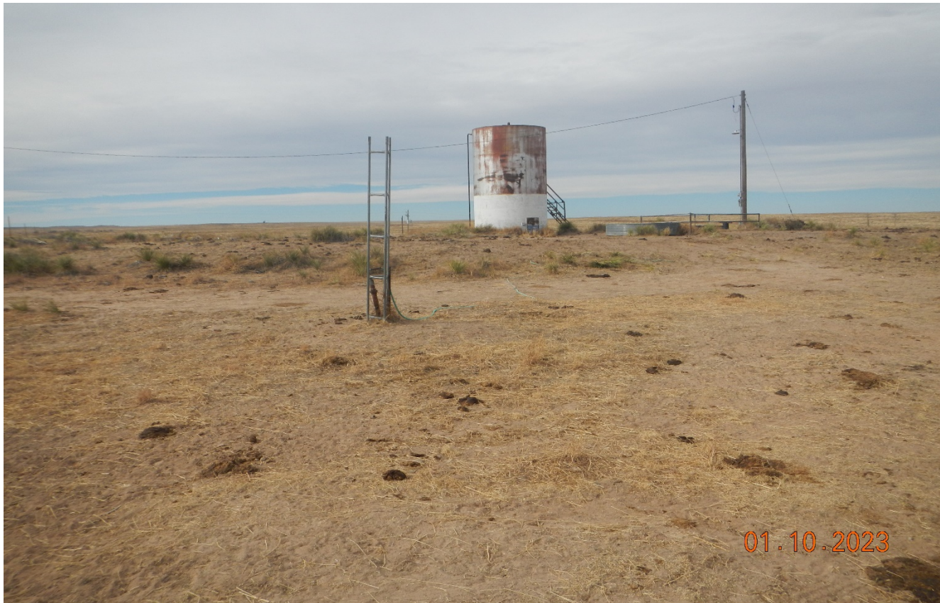
Photo 4. There is a permitted water well adjacent to the location and tank s not associated with the abandoned wellsite..
