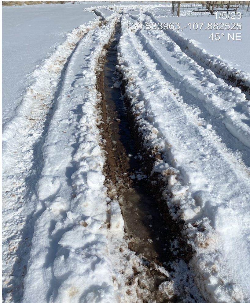
Photo 4. Photos show lack of stabilization/compaction at the upper/northern portion of the location.
