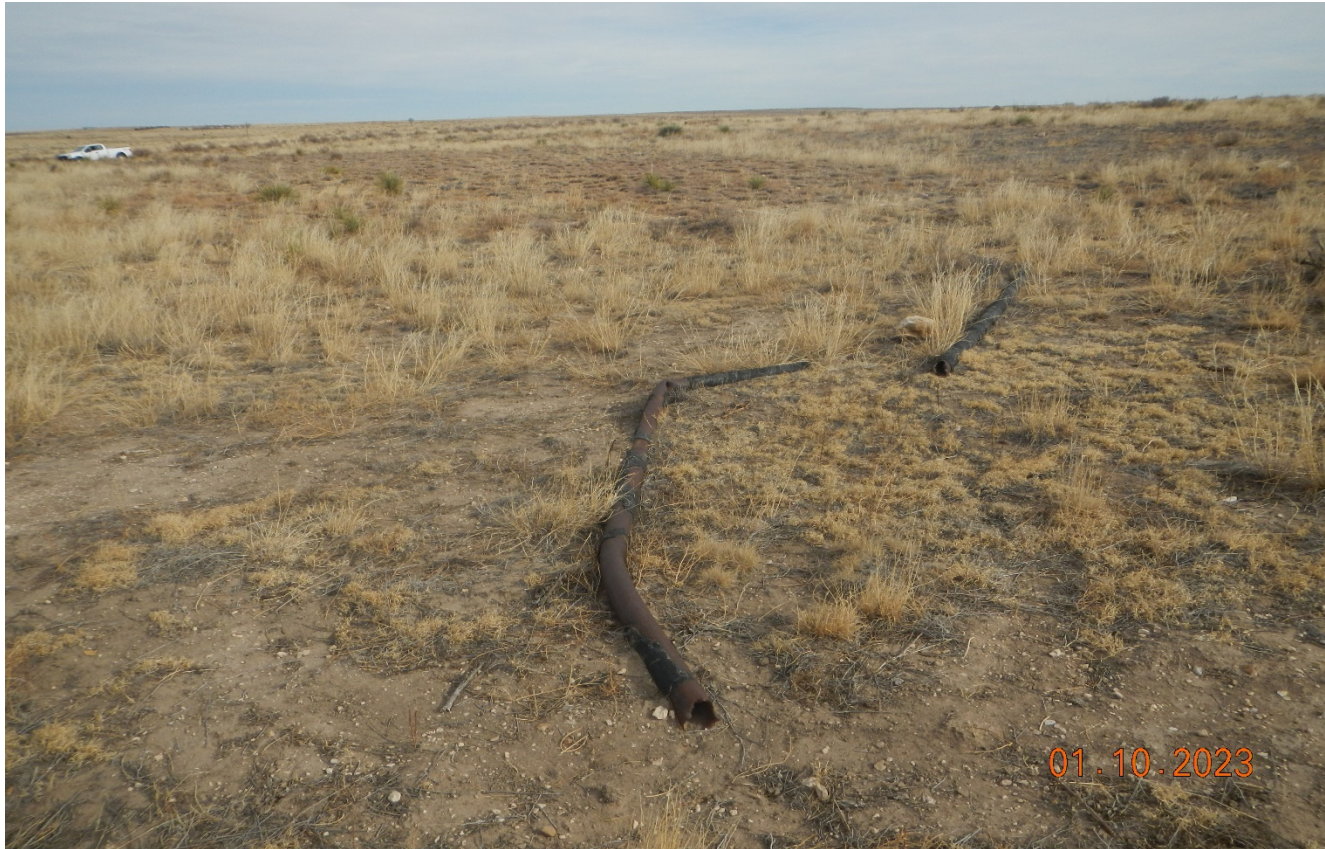
Photo 3. There are pieces of pipe that remain at south side of the location that need to be removed.
