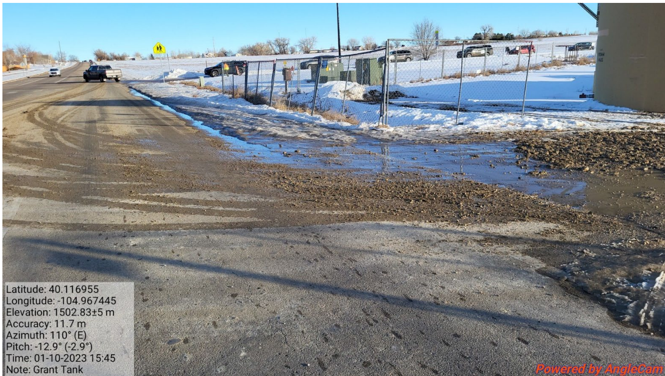
Photo 5 – Contractor Photo - 1/10/2023. Tracking observed on to Godding Hollow Pkwy. Tracking pad unmaintained.
