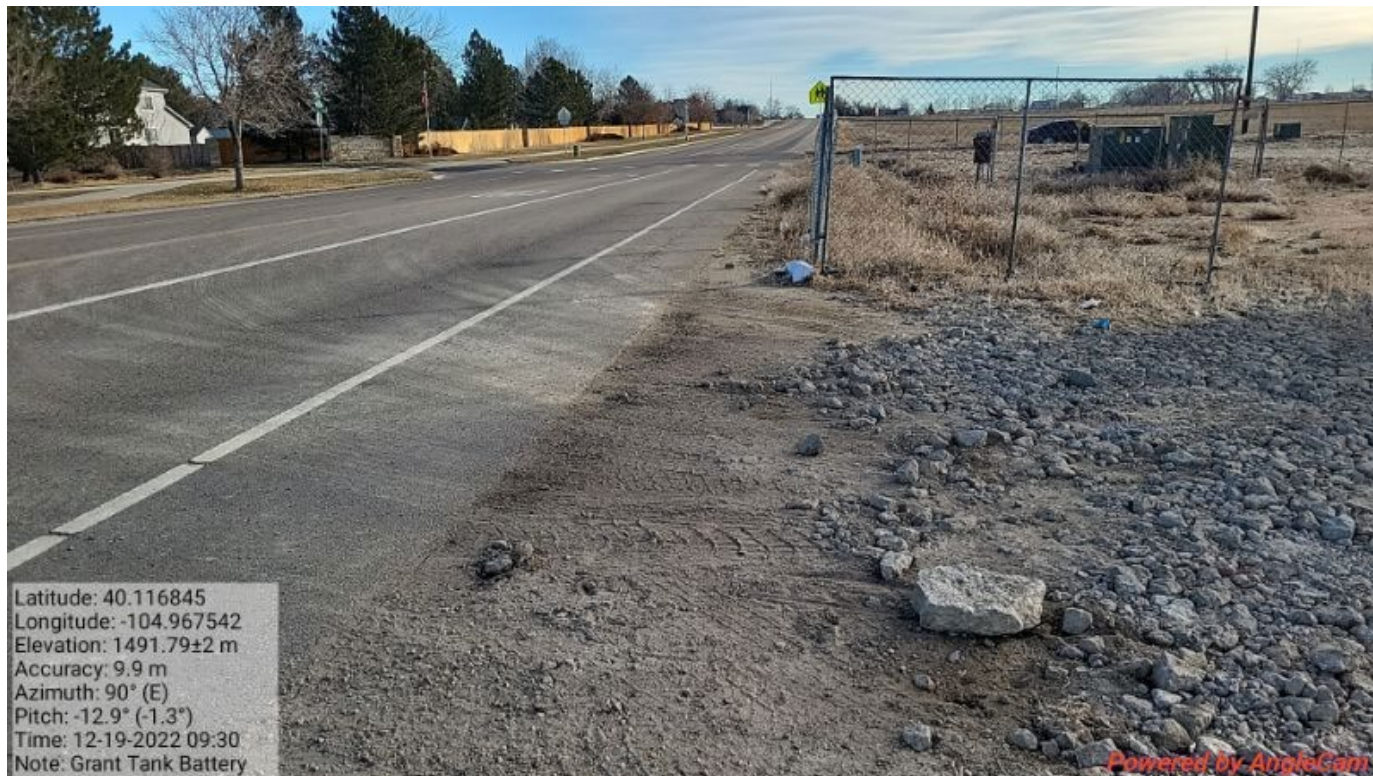
Photo 16 – Contractor Photo - 12/19/2022. Tracking observed on to Godding Hollow Pkwy.
