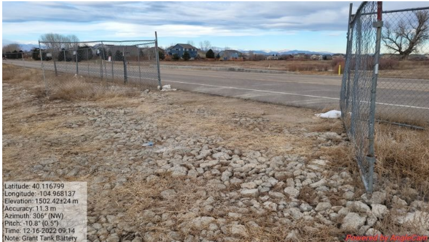
Photo 18 – Contractor Photo - 12/16/2022. Tracking observed on to Godding Hollow Pkwy. Tracking pad unmaintained.
