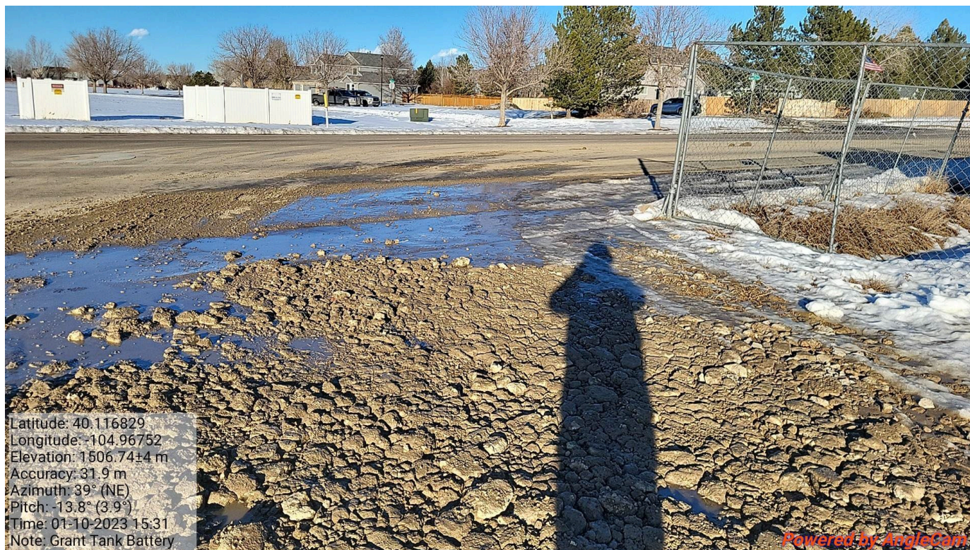
Photo 4 – Contractor Photo - 1/10/2023. Tracking observed on to Godding Hollow Pkwy. Tracking pad unmaintained.
