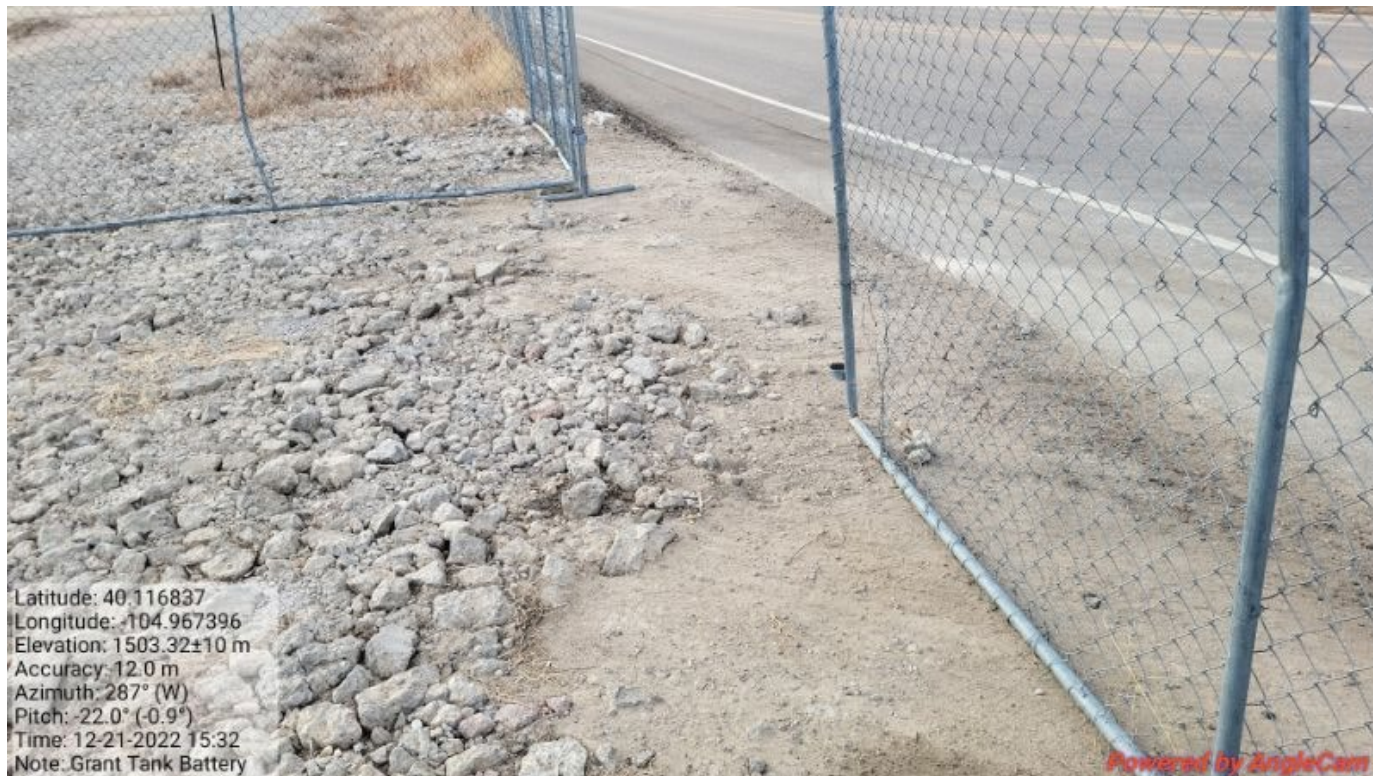
Photo 12 – Contractor Photo - 12/21/2022. Tracking pad unmaintained.
