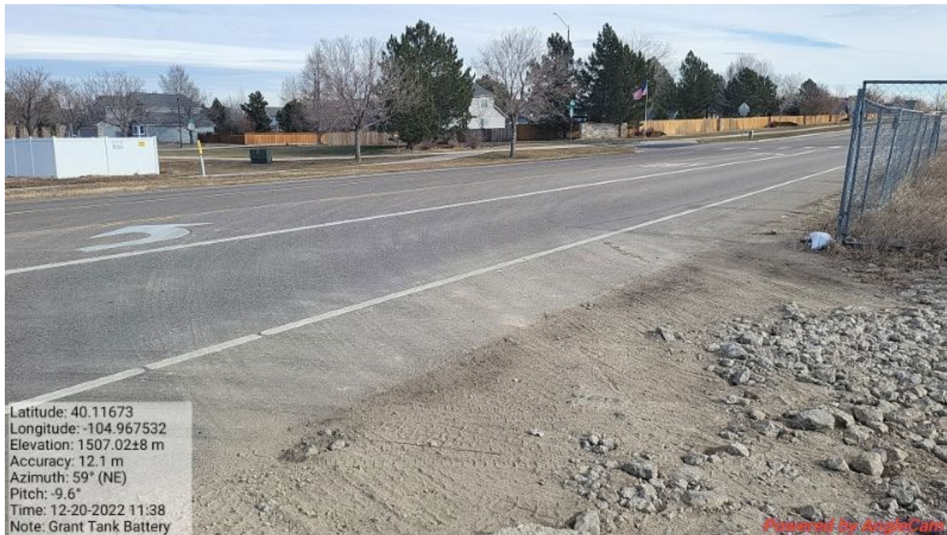
Photo 14 – Contractor Photo - 12/20/2022. Tracking observed on to Godding Hollow Pkwy.
