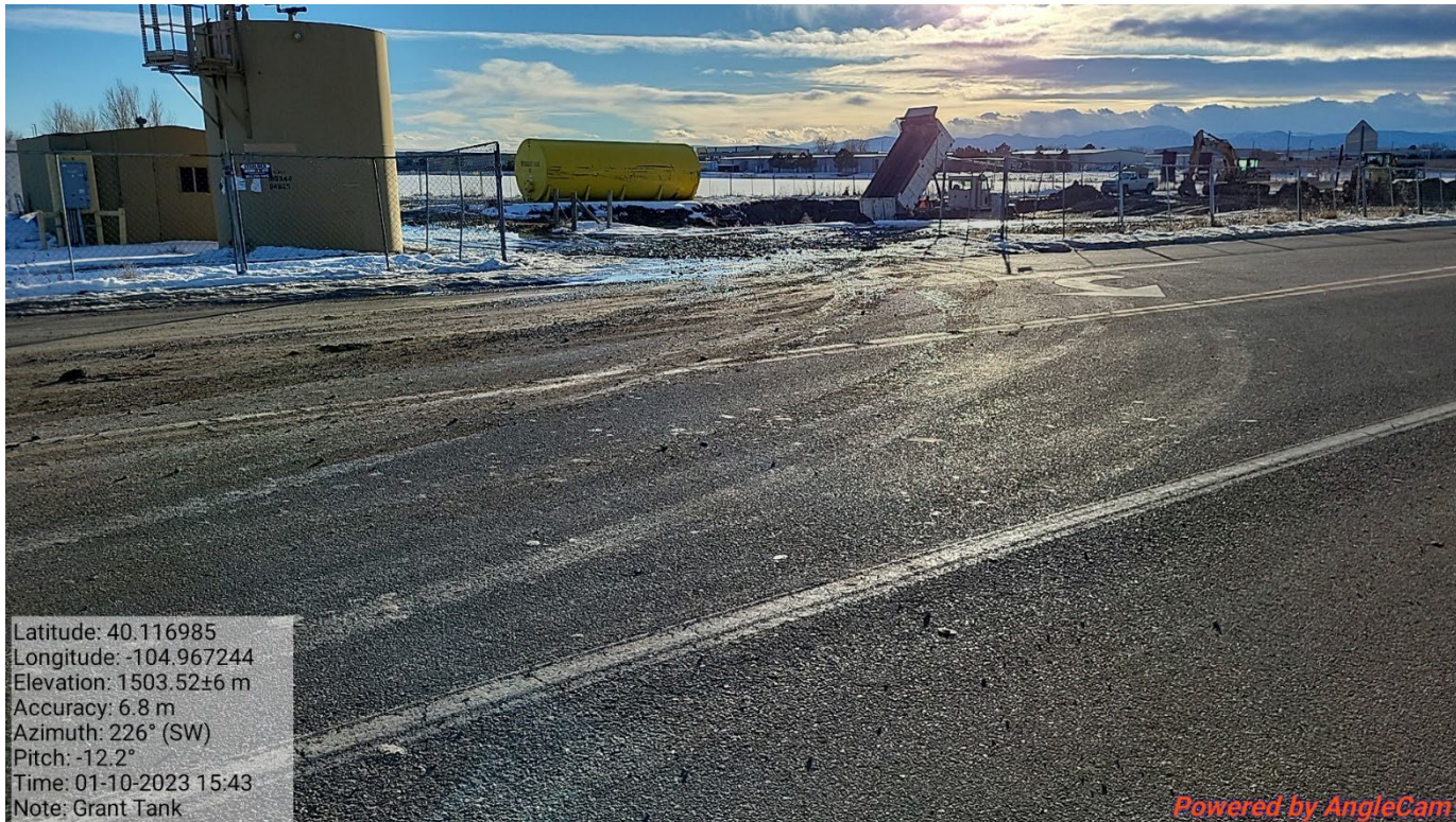
Photo 1 – Contractor Photo - 1/10/2023. Backfill in process. Tracking observed on to Godding Hollow Pkwy.
