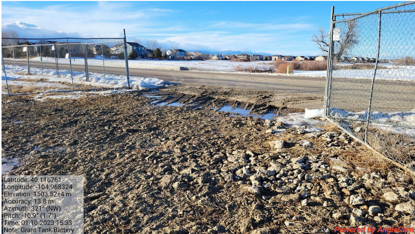
Photo 6 – Contractor Photo - 1/10/2023. Tracking observed on to Godding Hollow Pkwy. Tracking pad unmaintained.
