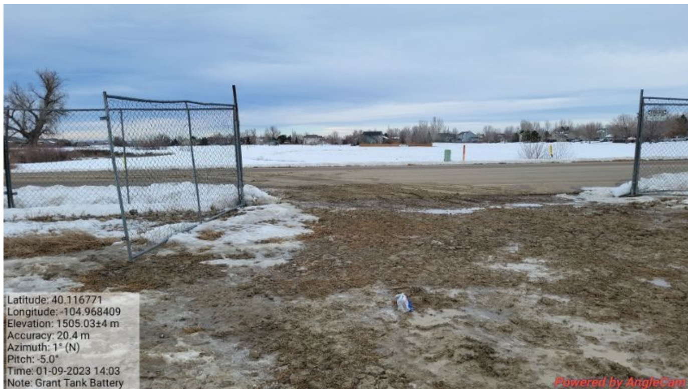
Photo 9 – Contractor Photo - 1/9/2023. Tracking observed on to Godding Hollow Pkwy. Tracking pad unmaintained.
