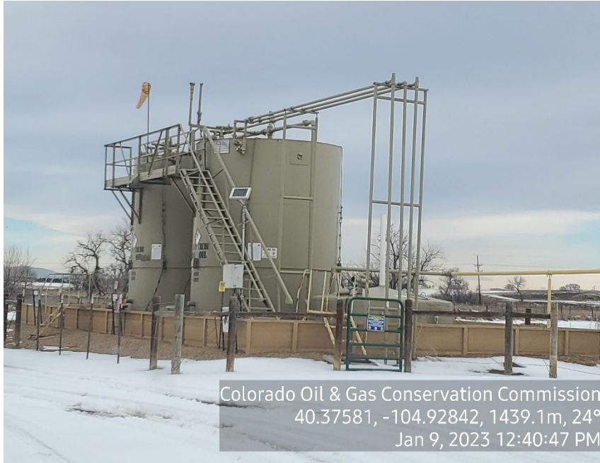
Photo 5: Centralized Tank Battery
