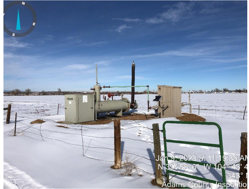
Photo# 2 SEPARATOR & METER.
