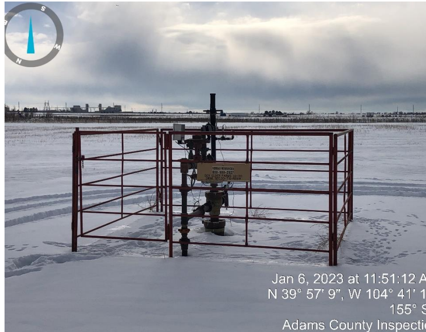
Photo# 3 Well Head.
