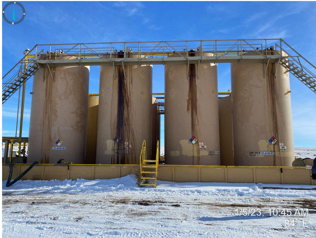
Photo 1. Facing east towards tank batteries. Photo illustrates crude released from thief hatches and dripping down the sides of the batteries.
