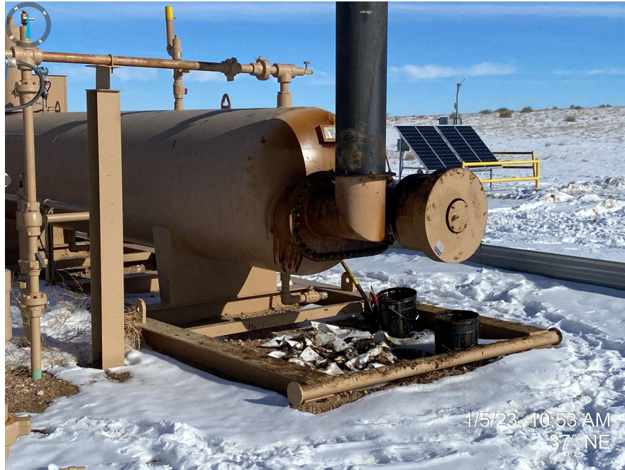
Photo 4. Facing northeast/northwest towards separator at the north end of the location. Photos illustrates a failed gasket that resulted in fluid exiting the equipment.
