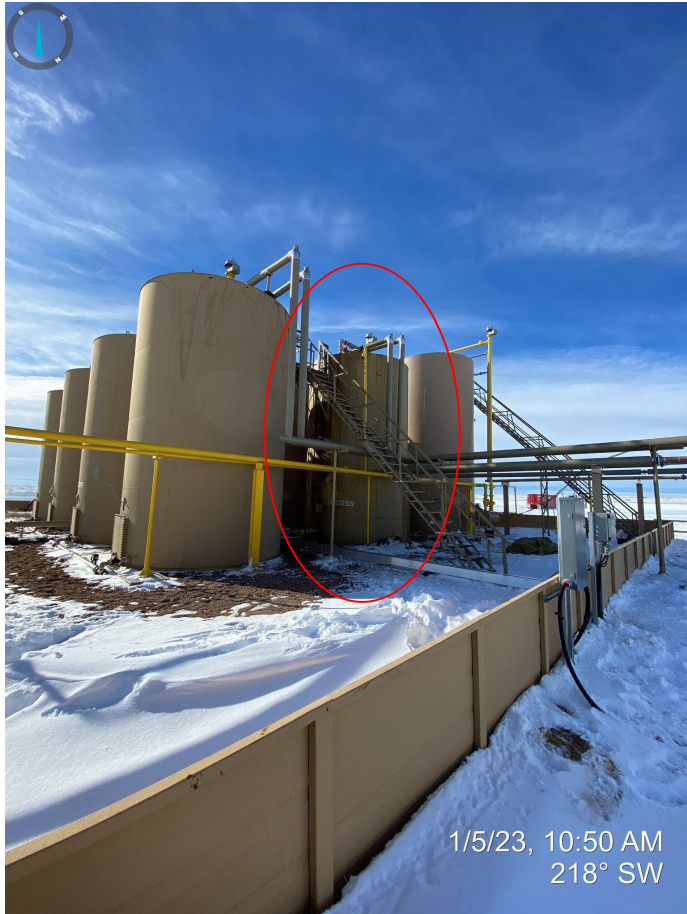
Photo 3. Facing southwest/south towards tank battery. Red outline shows crude spill on northern/middle tank.
