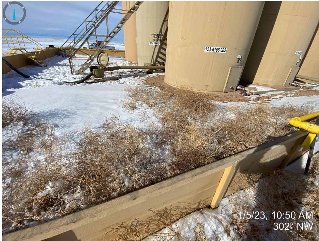
Photo 6. Facing northwest at tank battery. Photo illustrates tumbleweeds accumulated in and around equipment. This is considered debris, presents a potential fuel source for fire, and needs to be disposed of.
