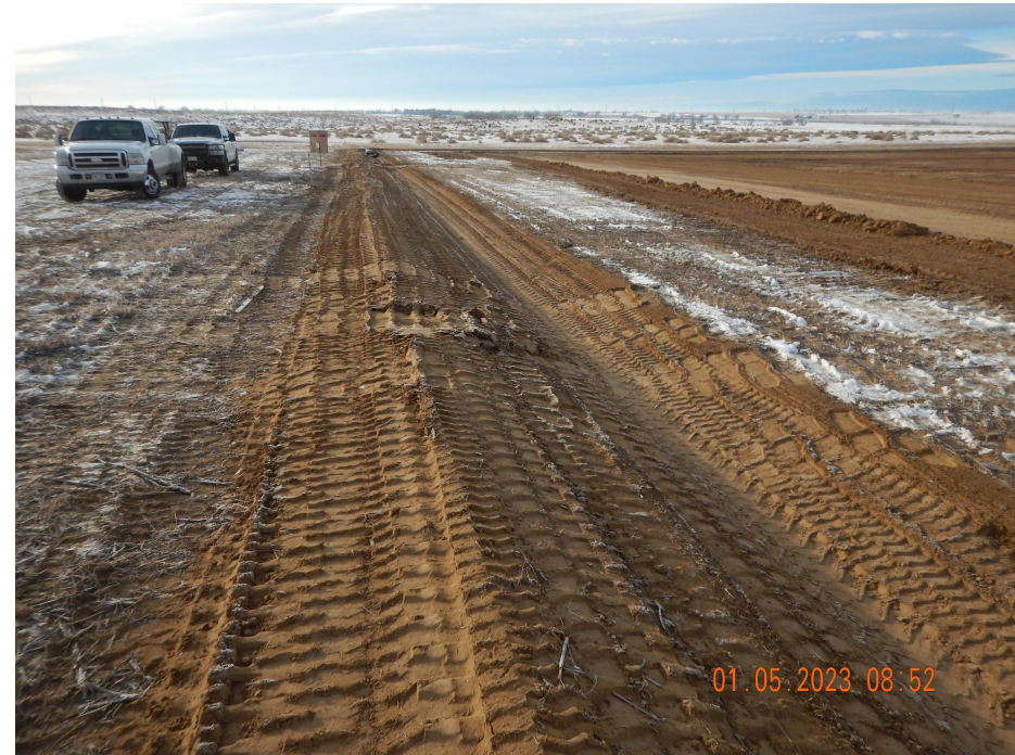
Photo 6. Photo taken from the eastern location, facing South. Photo illustrates a ditch and berm BMP installed around the entire perimeter of location during construction Operations.
