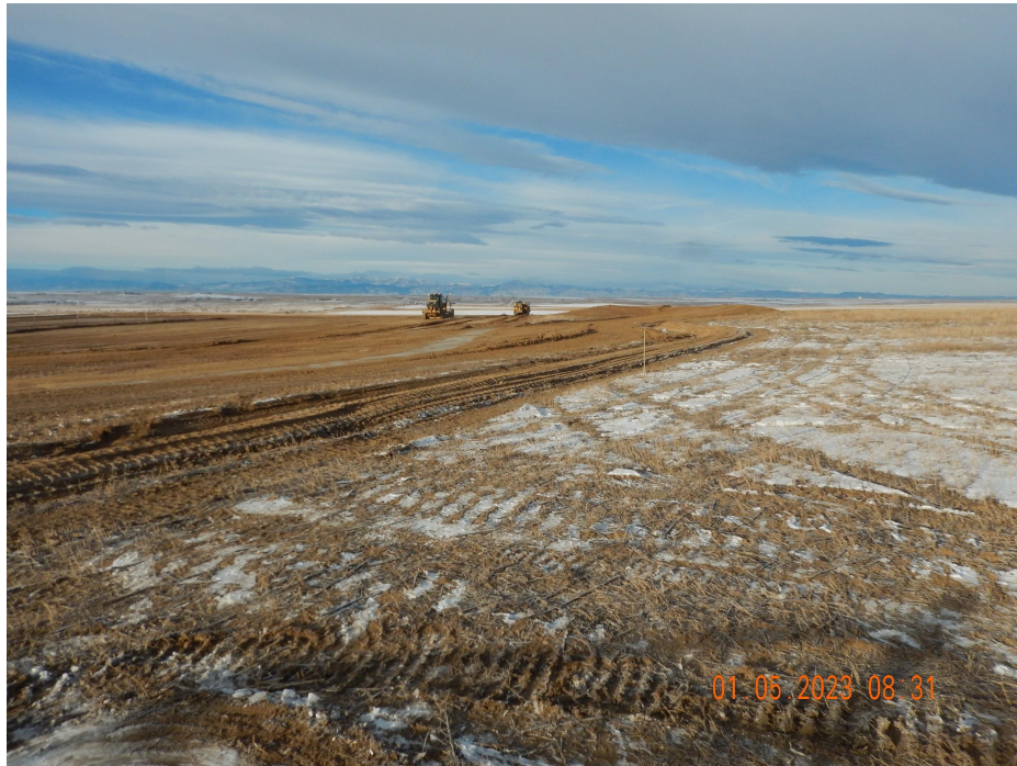
Photo 3. Photo taken from the northeastern location, facing West. Photo illustrates Operator is conducting topsoil salvage operations.
