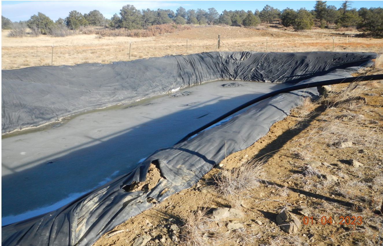
Photo 2. Facing toward the lined pit. The pit liner is torn in numerous places.
