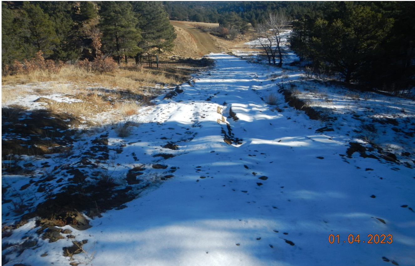
Photo 1. Facing northeast along the main road. There is erosion along this area of road that needs to be repaired.
