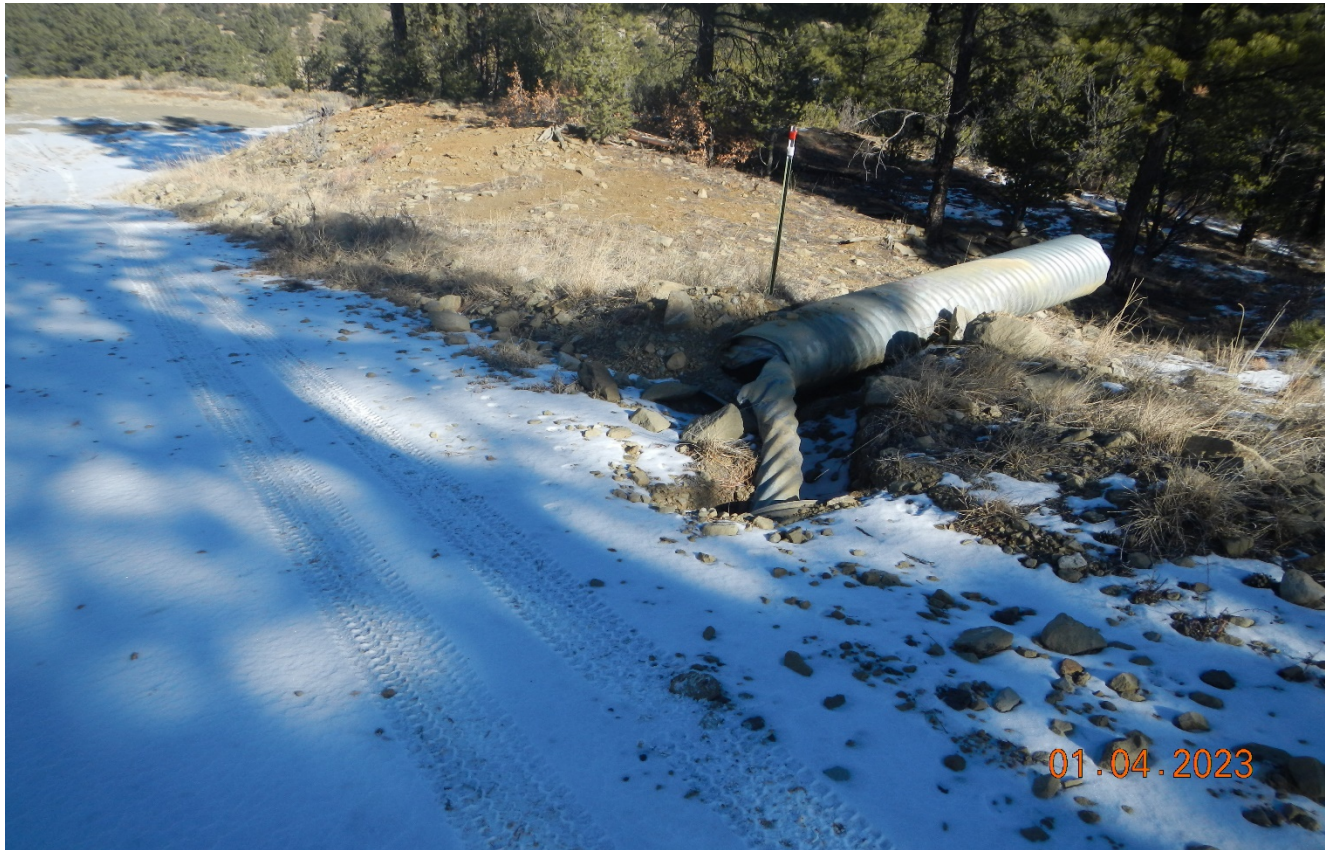
Photo 2. There is a damaged culvert near the location which should be cut off and armored with outlet protection.
